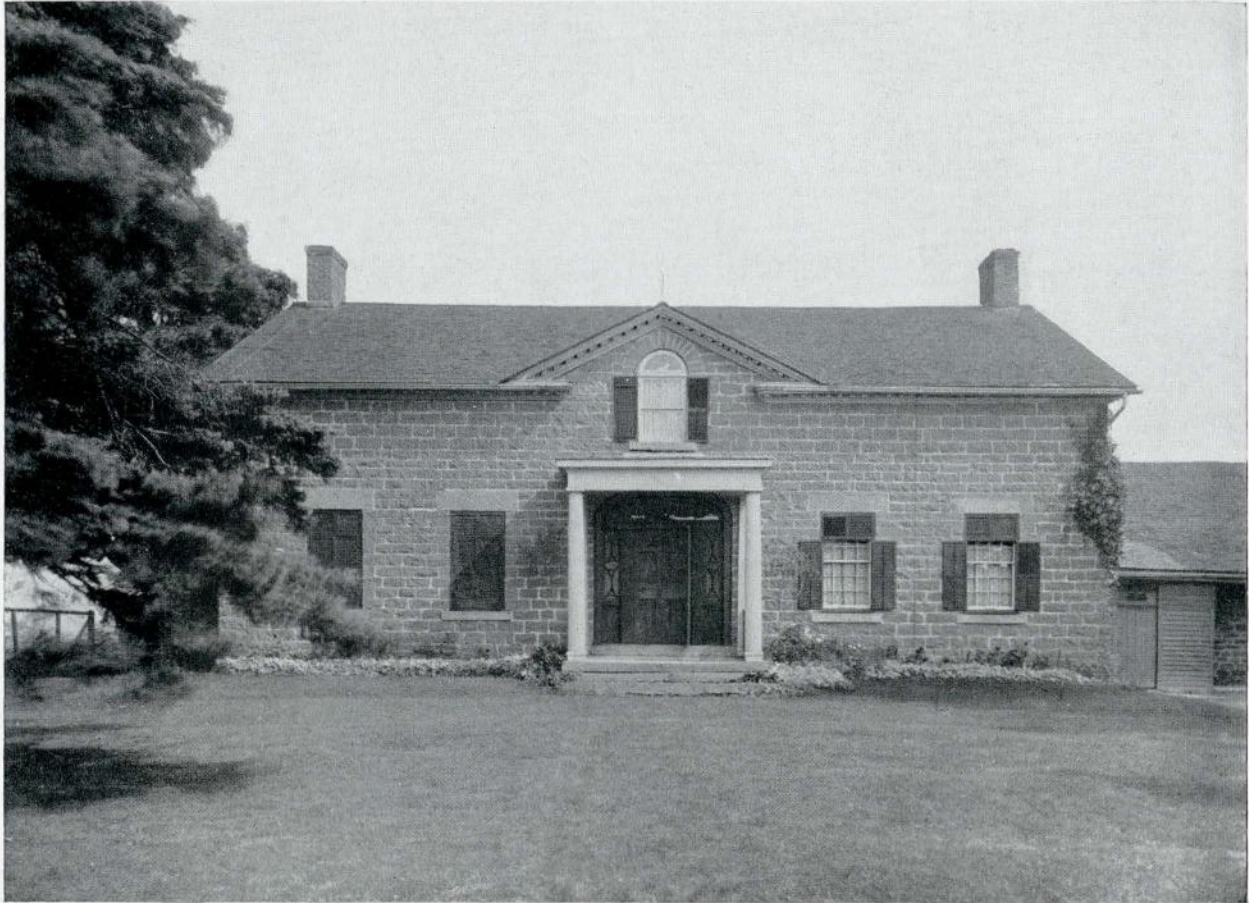
FIG. 7. BURNSIDE HOUSE, BROCKVILLE, ONTARIO
