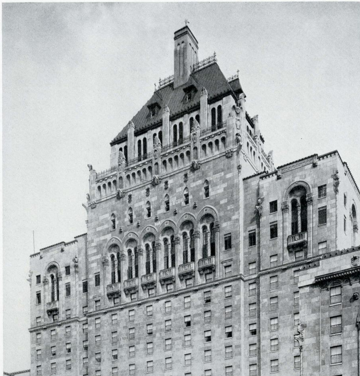
DETAIL OF TOWER
