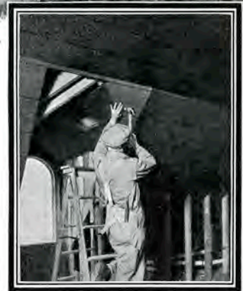
The cork-lined home of Mr. William P. Fosdick, Cincinnati, Ohio. Charles F. Cellarius, architect.
