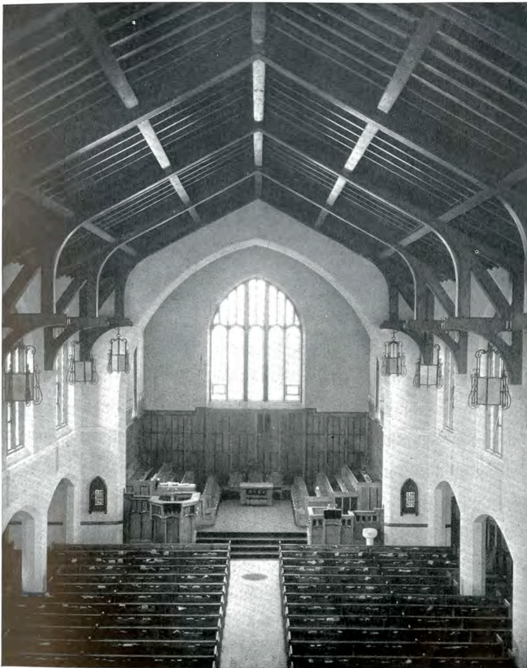
VIEW TOWARDS CHANCEL—ST. ANDREW'S UNITED CHURCH, HALIFAX, N.S. Wickson & Gregg, Architects; C. A. Fowler, Associate
