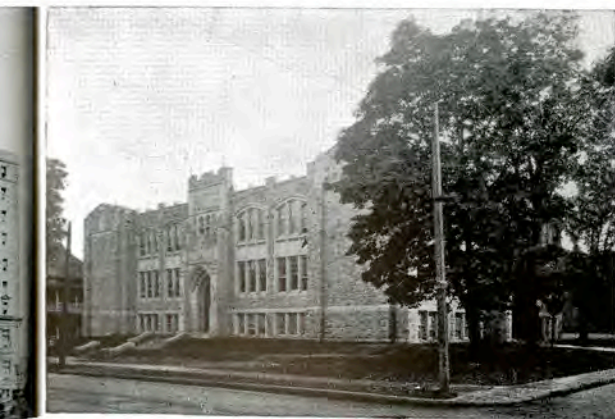
CATHOLIC CATHEDRAL HIGH SCHOOL , Hamilton, Ont. 1 3/4" First Grade Maple
