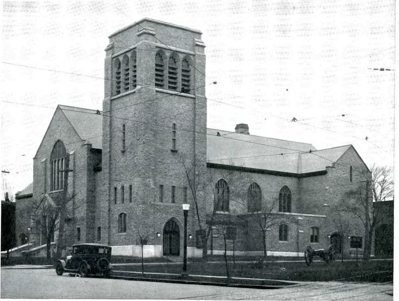
ST. ANDREW'S UNITED CHURCH, HALIFAX, N.S. Wickson & Gregg, Architects; C. A. Fowler, Associate
