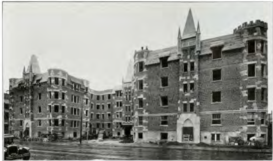
"Garden Court," Durocher and Bernard Streets, Montreal, Que. Entire 40 suites equipped with Frigidaire. Architects, Perrault & Gadbois, Montreal.
