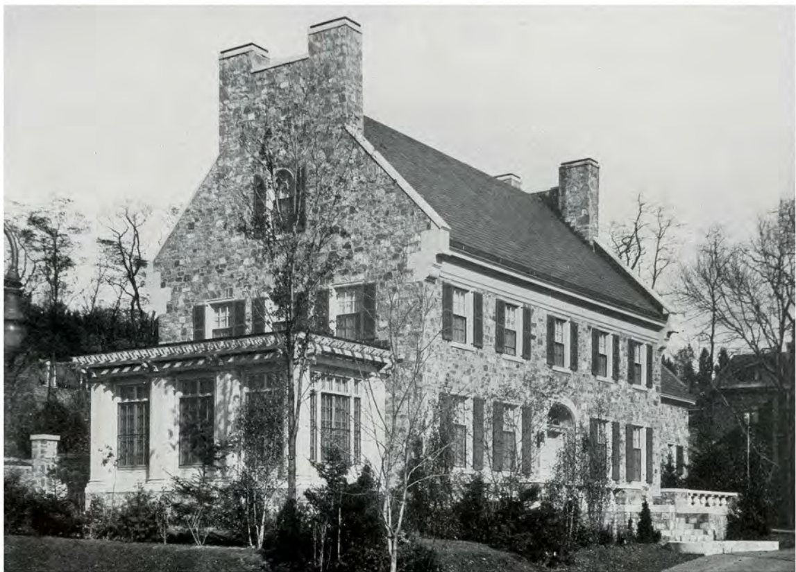
RESIDENCE OF A. J. NESBITT, FORDEN CRESCENT, WESTMOUNT, P.Q. Shorey & Ritchie, Architects
