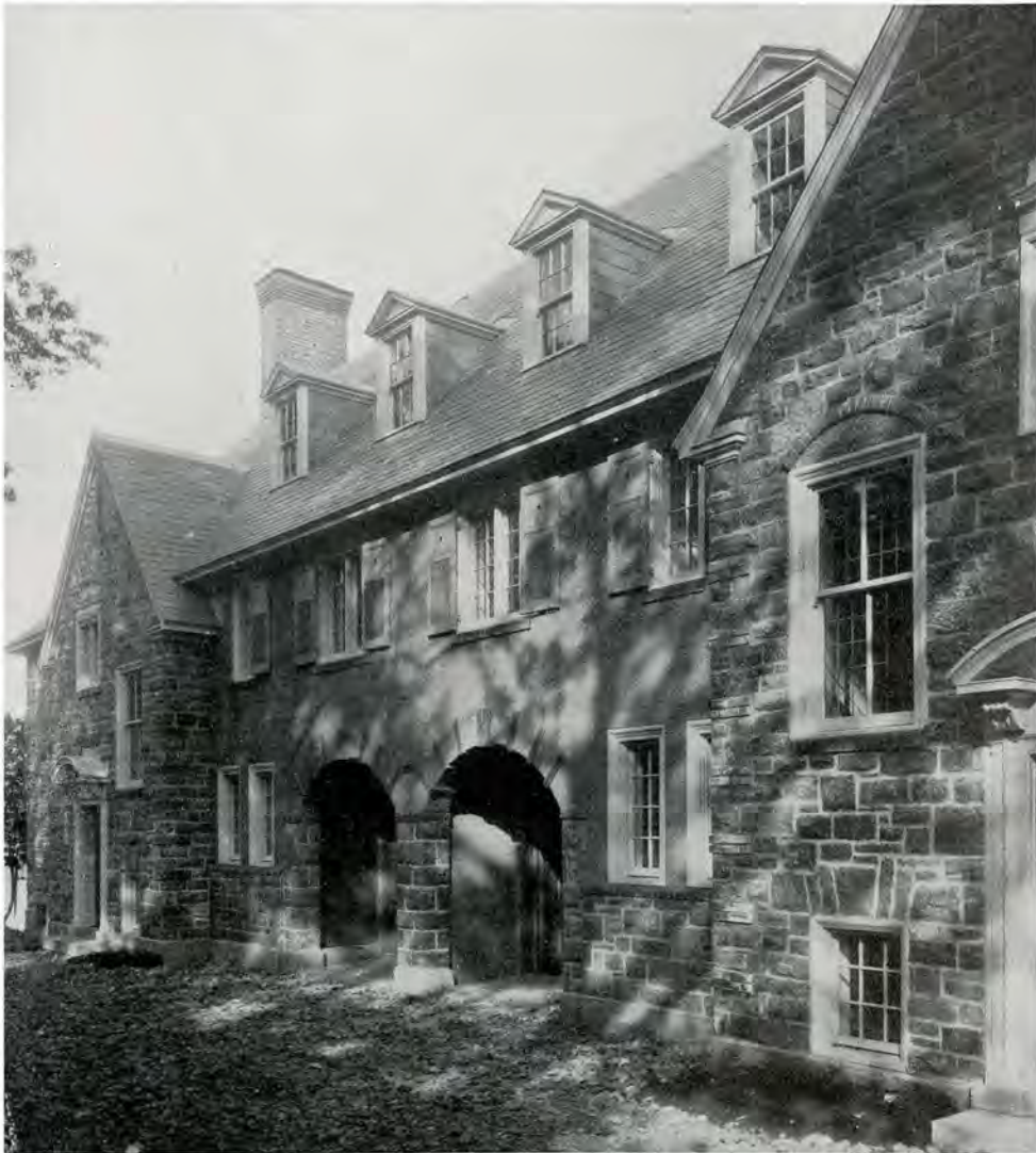
SEMI-DETACHED HOUSES, BELVEDERE PLACE, WESTMOUNT, P.Q., FOR W. M. AND J. H. BIRKS, ESQS. Nobbs & Hyde, Architects
