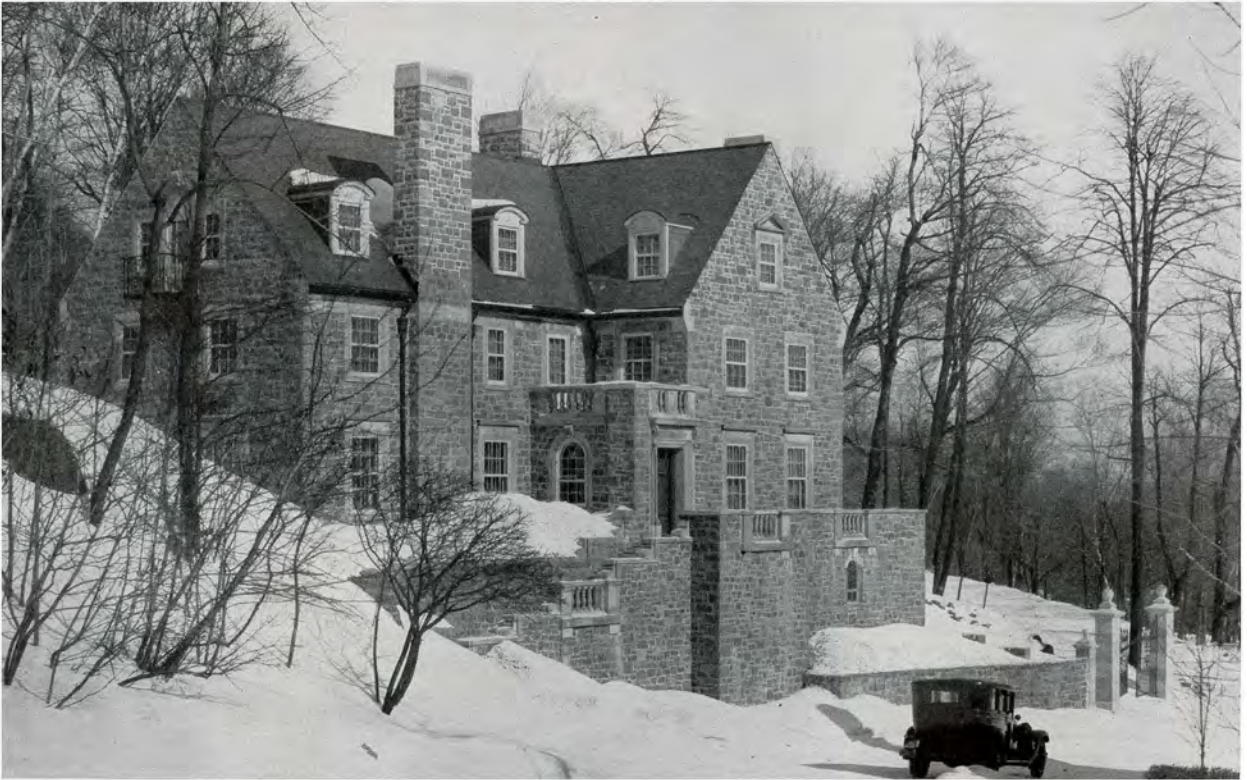
RESIDENCE OF W. R. G. HOLT, ESQ., REDPATH CRESCENT, MONTREAL H. L. Fetherstonhaugh, A.R.I.B.A., Architect
