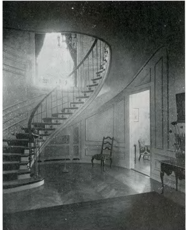
MAIN STAIRWAY, RESIDENCE OF T. S. GILLESPIE, ESQ. Barott & Blackadder, Architects
