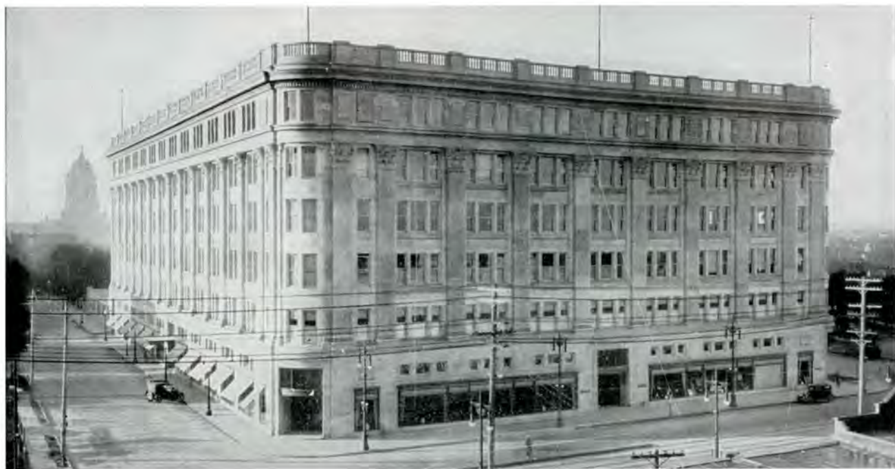
Constructed in the winter: Hudson's Bay Company Store, Winnipeg
