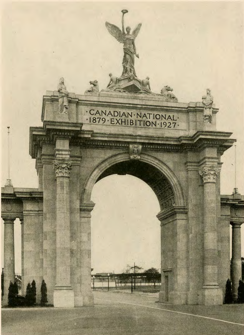
CENTRAL ARCHWAY—THE PRINCES' GATES, CANADIAN NATIONAL EXHIBITION Chapman and Ozley, Architects
