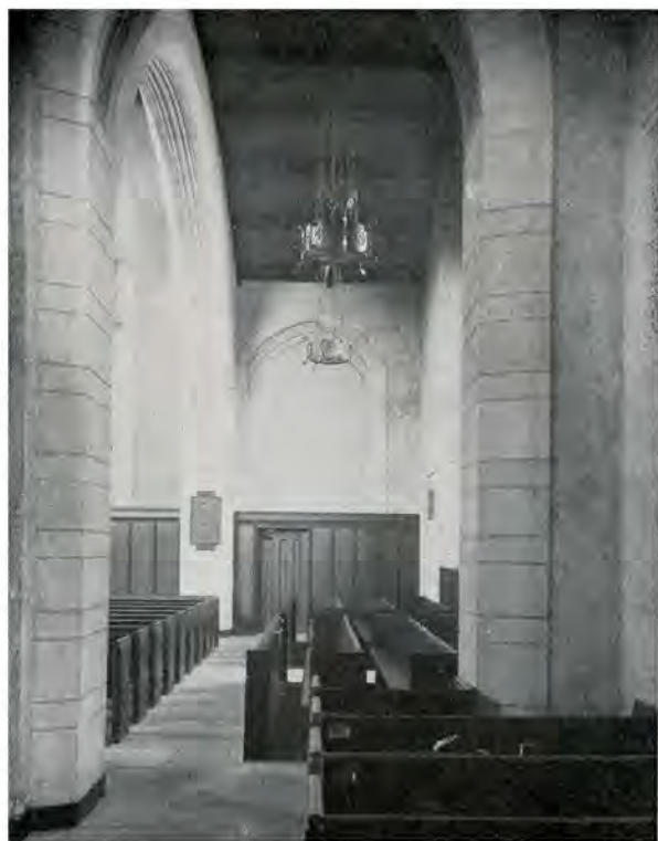
DOMINION-DOUGLAS CHURCH, WESTMOUNT, P. Q. NORTH TRANSEPT LOOKING WEST FROM NORTH AISLE
