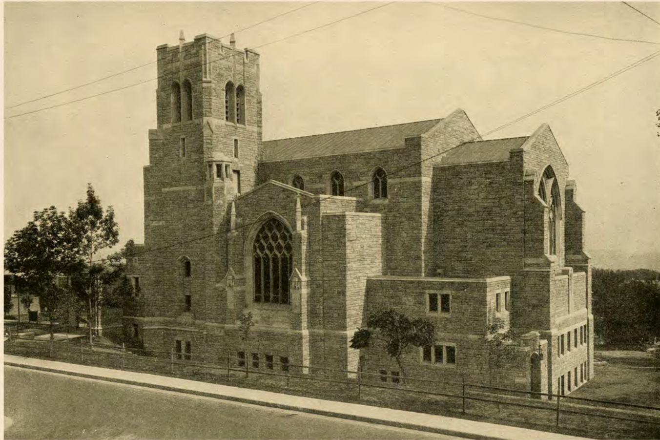
DOMINION-DOUGLAS CHURCH, WESTMOUNT, P. Q.—FROM THE NORTH-WEST Hugh G. Jones, Architect
