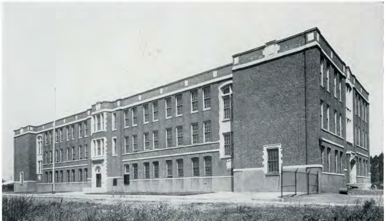
CONNAUGHT SCHOOL, MONTREAL, P.Q. John S. Archibald, Architect
