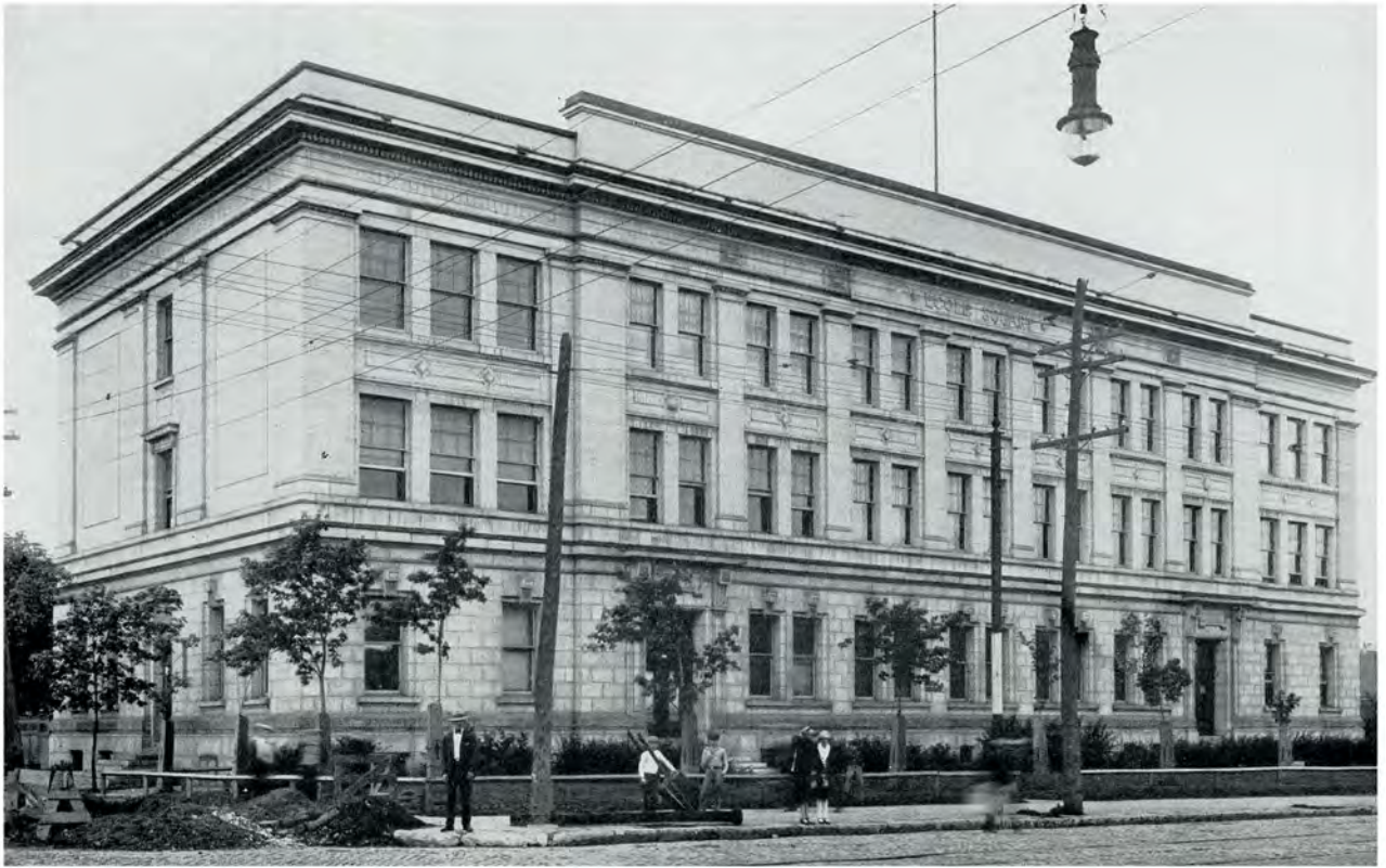
SOUART SCHOOL, PAPINEAU AVENUE, MONTREAL, P.Q. J. O. Marchand, Architect
