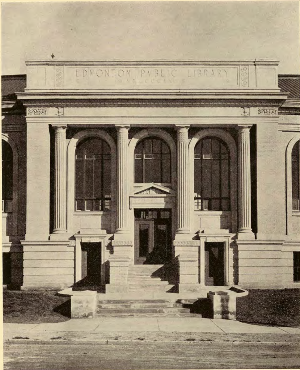
DETAIL OF ENTRANCE, EDMONTON PUBLIC LIBRARY
