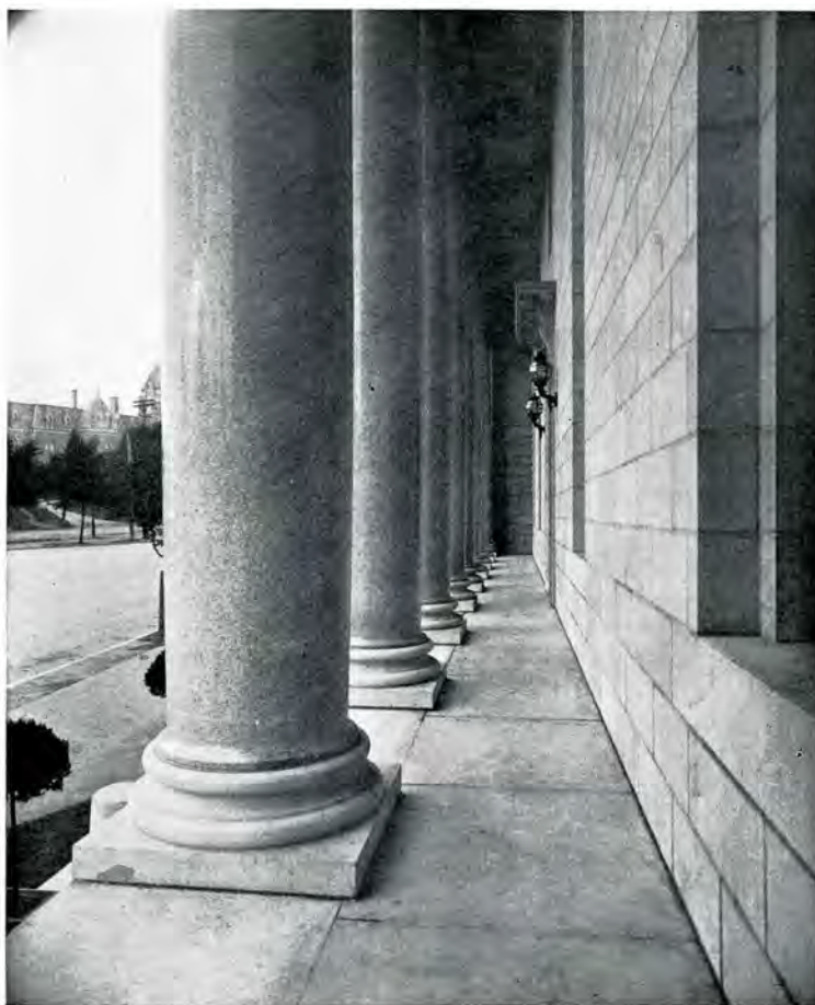
DETAIL OF FACADE, THE LIBRARY OF THE CITY OF MONTREAL
