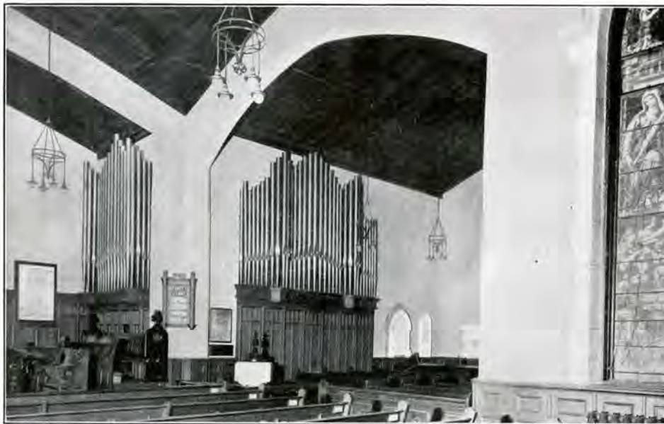
Interior of St. George's Church, St. Catharines, Ont. Walls finished in cream colored Morene, stippled and over-trowelled. The excellent reproduction of limestone around the windows is also Morene.
