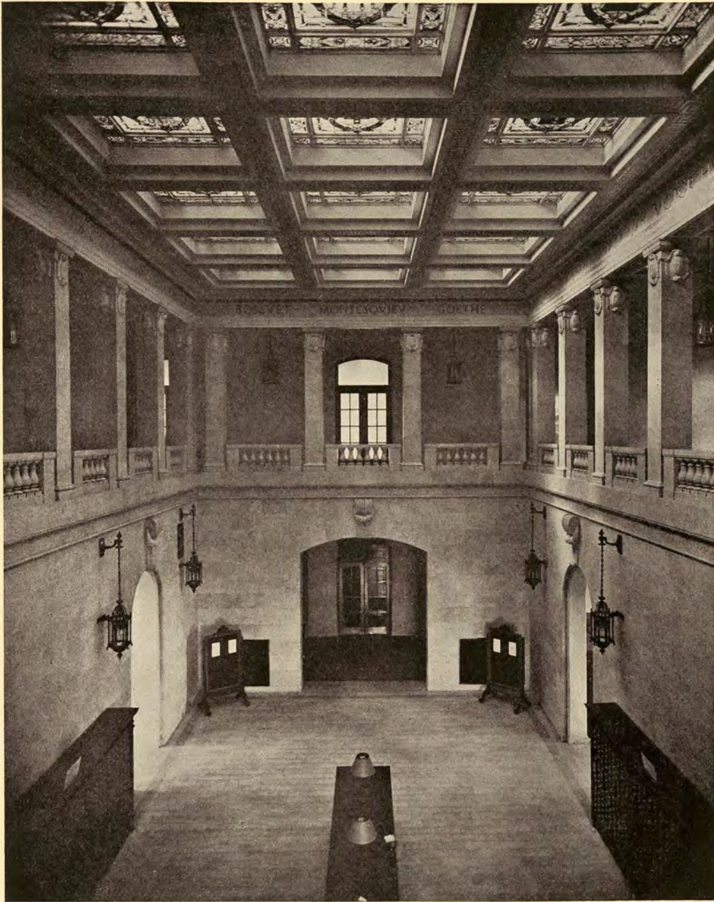
DISTRIBUTING HALL, THE LIBRARY OF THE CITY OF MONTREAL Eugène Payette, Architect
