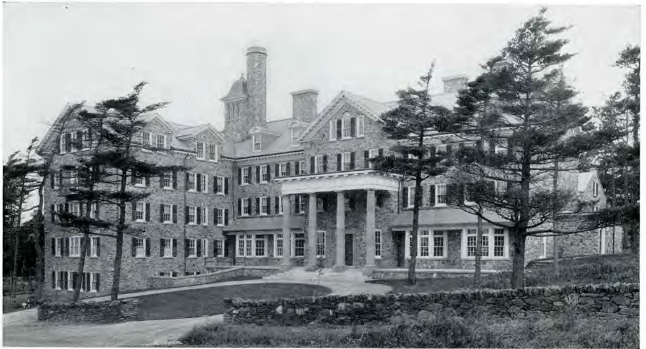
SHIRREFF HALL—WOMEN'S RESIDENCE, DALHOUSIE UNIVERSITY, HALIFAX, N.S. F. Darling, R.A.I.C., Consulting Architect.
