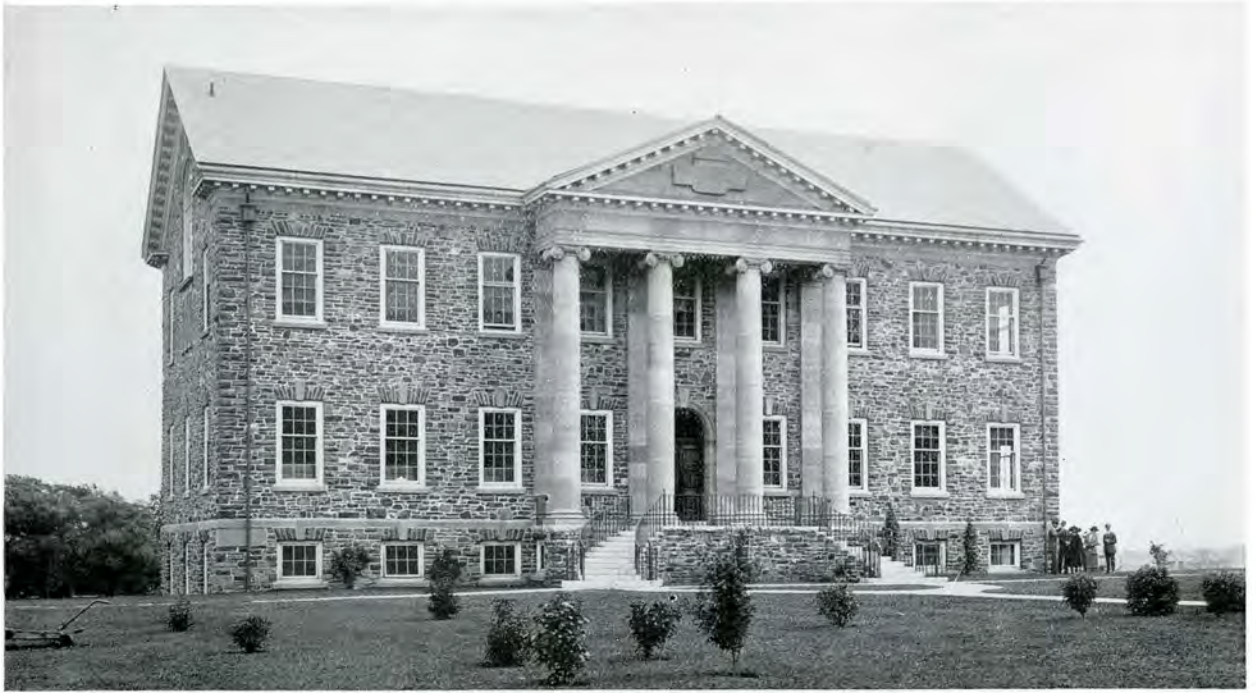
LAW BUILDING (at present used as Arts Building), DALHOUSIE UNIVERSITY, HALIFAX, N.S. A. R. Cobb, Architect. F. Darling, R.A.I.C., Consulting Architects.
