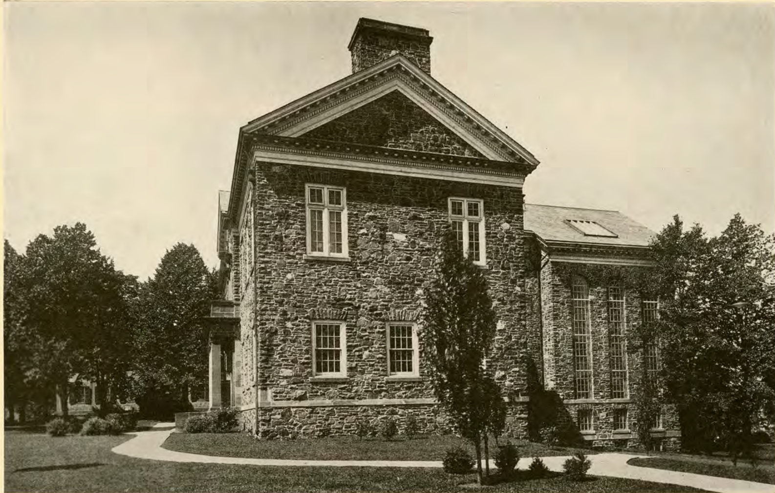
MACDONALD MEMORIAL LIBRARY, SHOWING STACK, DALHOUSIE UNIVERSITY, HALIFAX, N.S. A. R. Cobb, Architect. Frank Darling, R.A.I.C., Consulting Architect.
