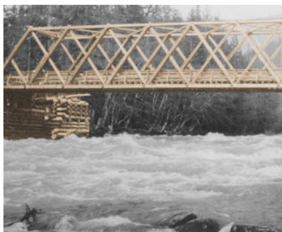
Timber cribbing foundation for bridge. District of Squamish Archives
