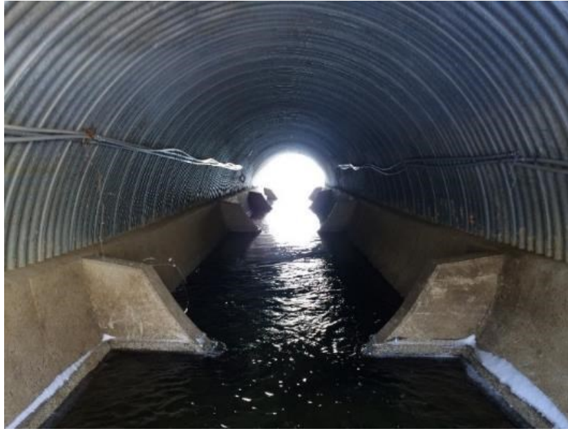
Figure 1.5 CMP culvert rehabilitated by the in-place installation of a concrete invert.
