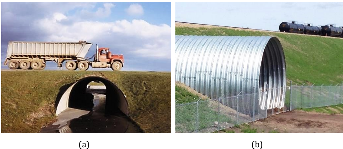
Figure 1.1 Typical culvert applications: a) highway culvert for stream crossing (Contech, 2017); and b) railroad culvert for small vehicle access (Armtec, 2015)
