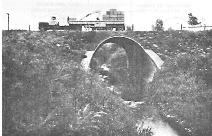
Figure 2.10 White Ash Creek culvert during live load testing (Bakht, 1980)
