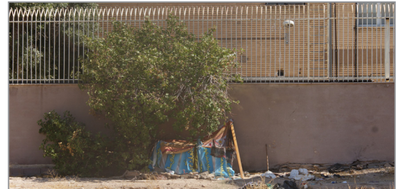
Figure 13: The area is not well maintained
