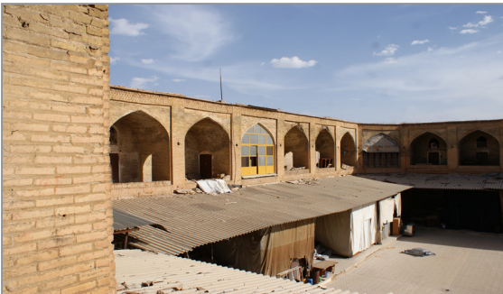
Figure 10: A deteriorating caravanserai used for storage in Zand complex
