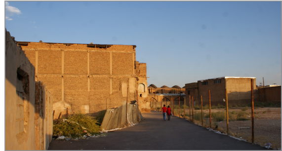
Figure 12: Deteriorating condition and poor circulation throughout Zand complex
