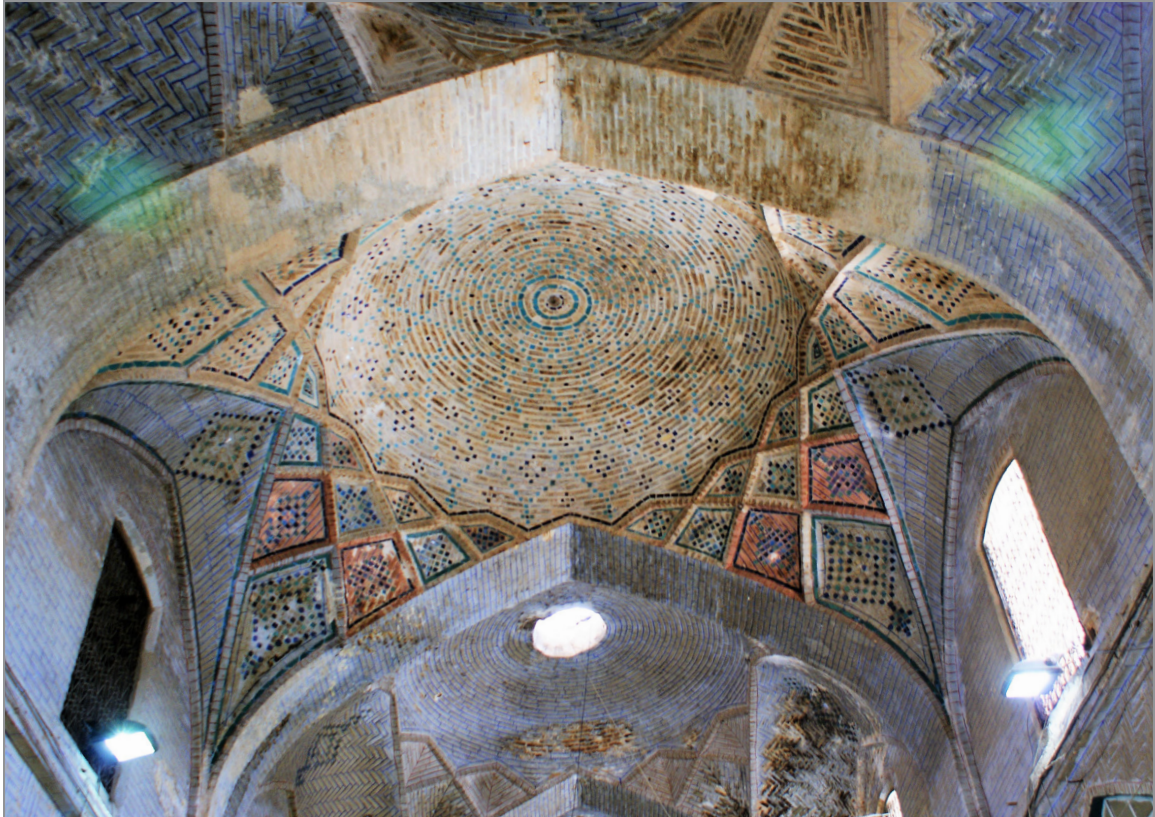
Figure 56: Zand complex bazaar ceiling geometry
