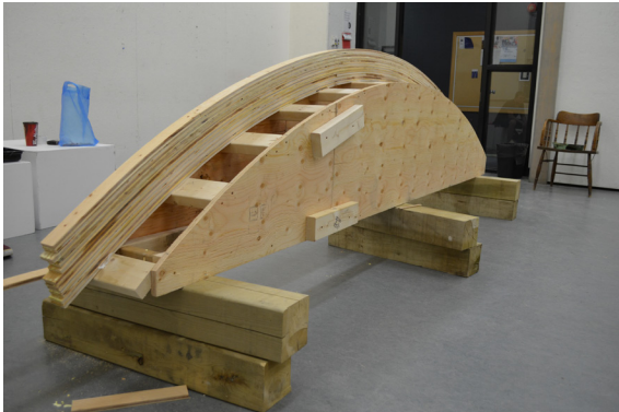
Formwork for all 3 bent glulams.
