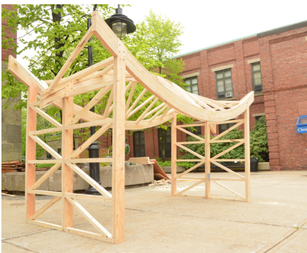
One structural bay of the glulam structure detail.
