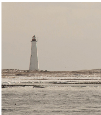
Figure 1 Cape Sable Lighthouse
