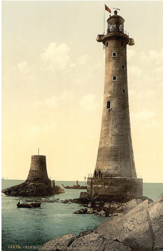
Figure 40 Smeaton's foundation remains standing next to the new light, (Matthews, 1978)
