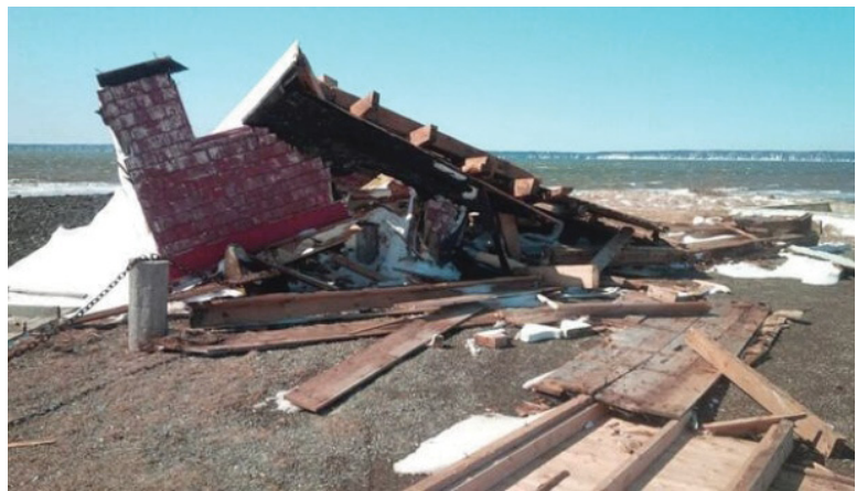
Figures 16-17 Images depicting the 140 year old wooden Church Point lighthouse before and after a spring storm in the southwestern part of Nova Scotia, (Robichaud, 2014)
