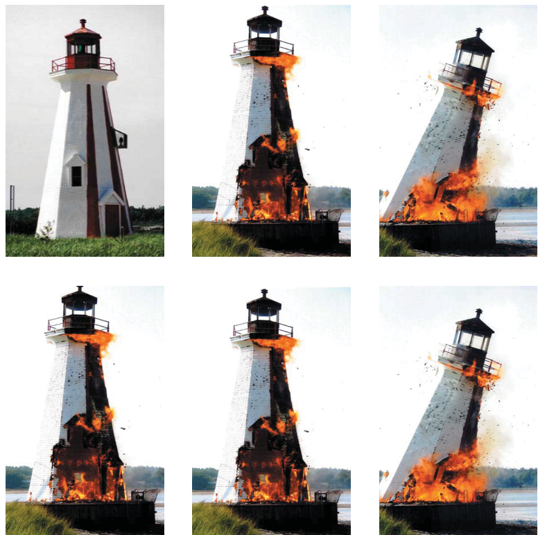
Figure 62 Fire destroying wood lighthouse at Pictou Bar - 2004, (Irwin, 2004)
