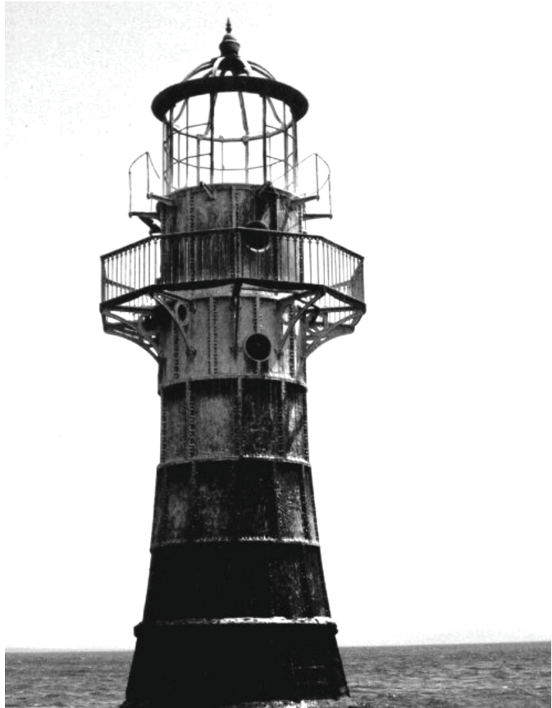
Figure 56 Whitford lighthouse steel structure, (Emmanuel, 1985)
