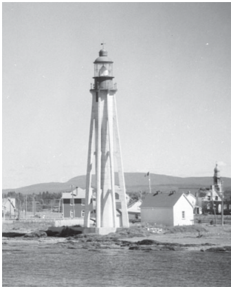
Figure 65 Flying buttress concrete lighthouse (Johnston, 1933)
