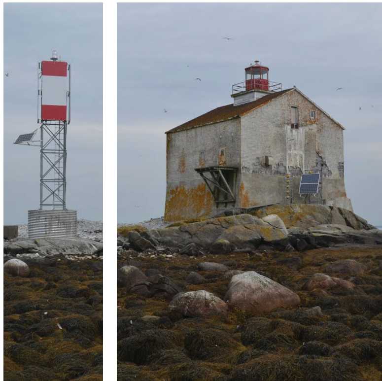
Figure 58 The Salvages lighthouse established in 1965 and neighbouring skeleton tower built in 2014, (The Salvages, 2016)
