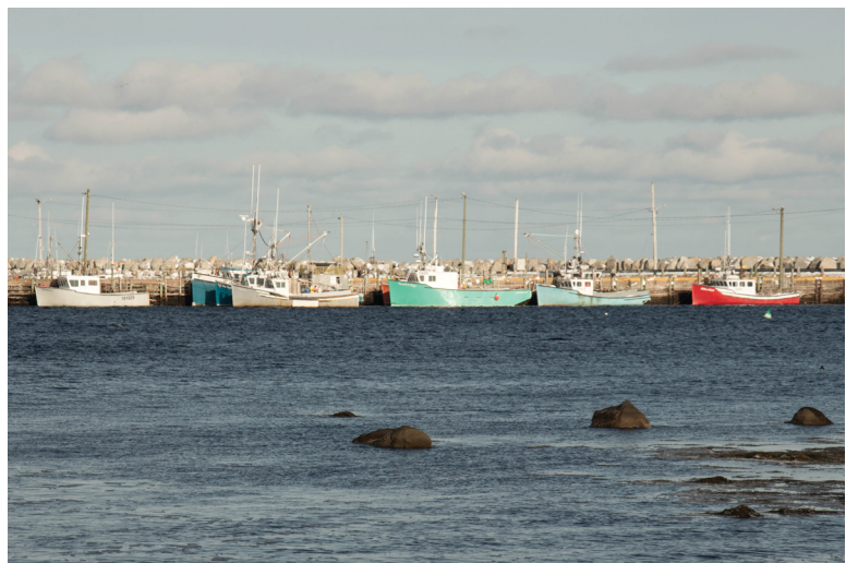
Figure 37 Government wharf in Port Mouton protected by a breakwater
