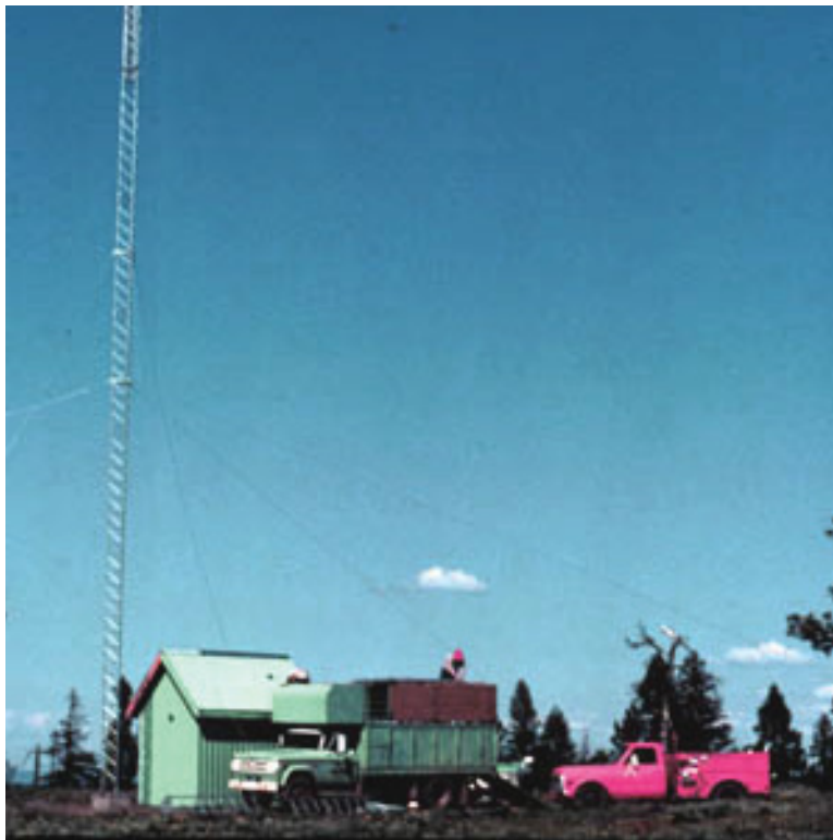
Figure 12 Image of an eLoran Tower during construction, (Loran Tower, 2001)
