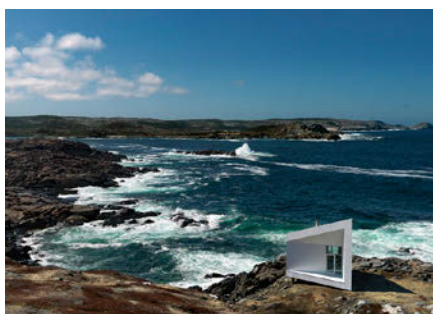
Fogo Island architecture by Todd Saunders. Nature highlighted by framed viewports. Photos by Bent René Synnevang.
