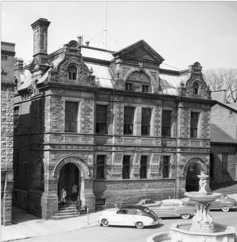
FIG. 1. FORMER BROCKVILLE POST OFFICE, COURTHOUSE AVENUE, BROCKVILLE, ONTARIO, 1882–1886. | GEORGE ELAND, C. 1950, FROM THE ARCHIVES OF THE BROCKVILLE MUSEUM.
