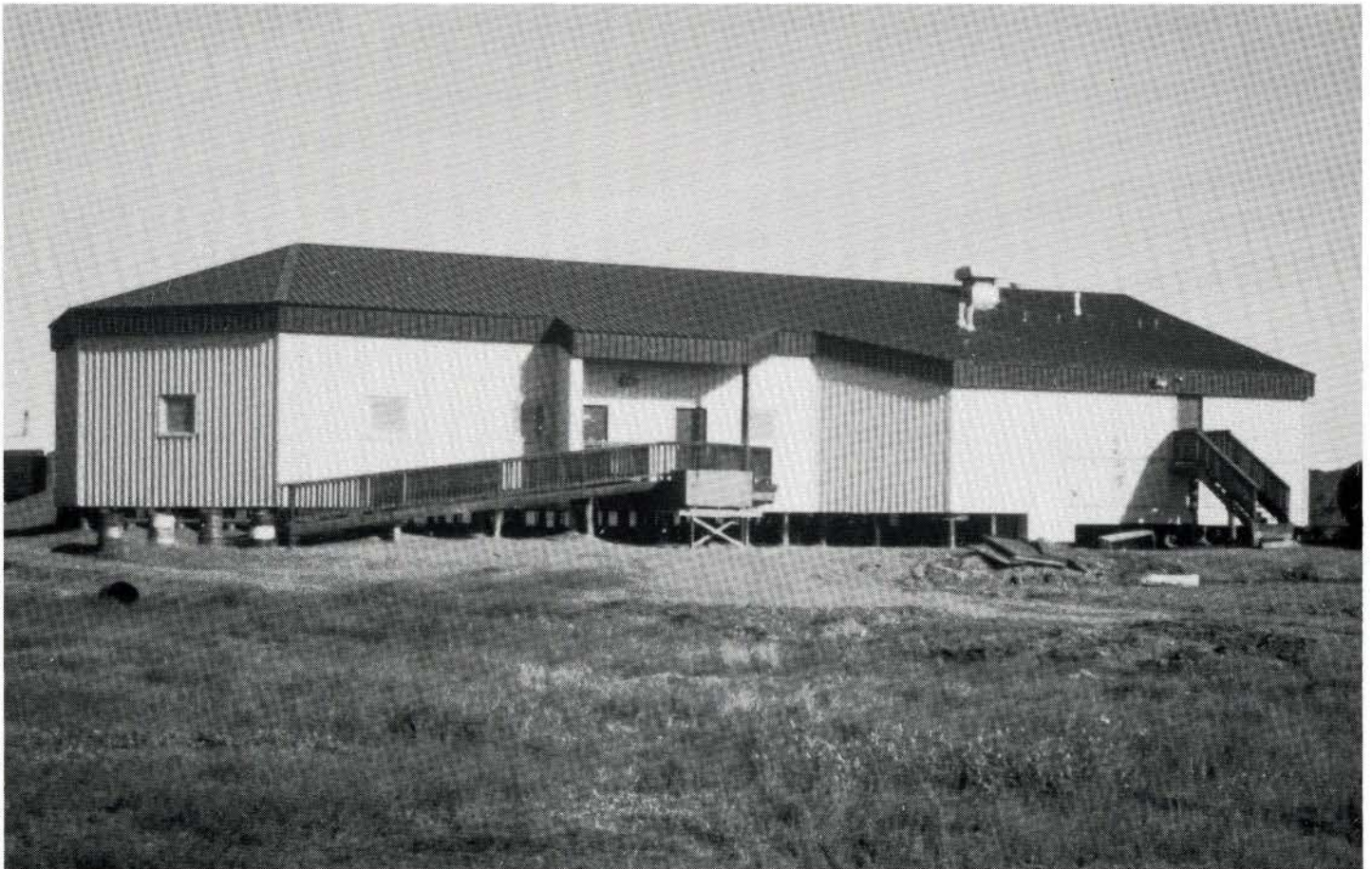
Figure 6. Tuktoyaktuk Community Centre, Tuktoyaktuk, NWT (1983). Exterior showing roof and door form for clearing snow.
