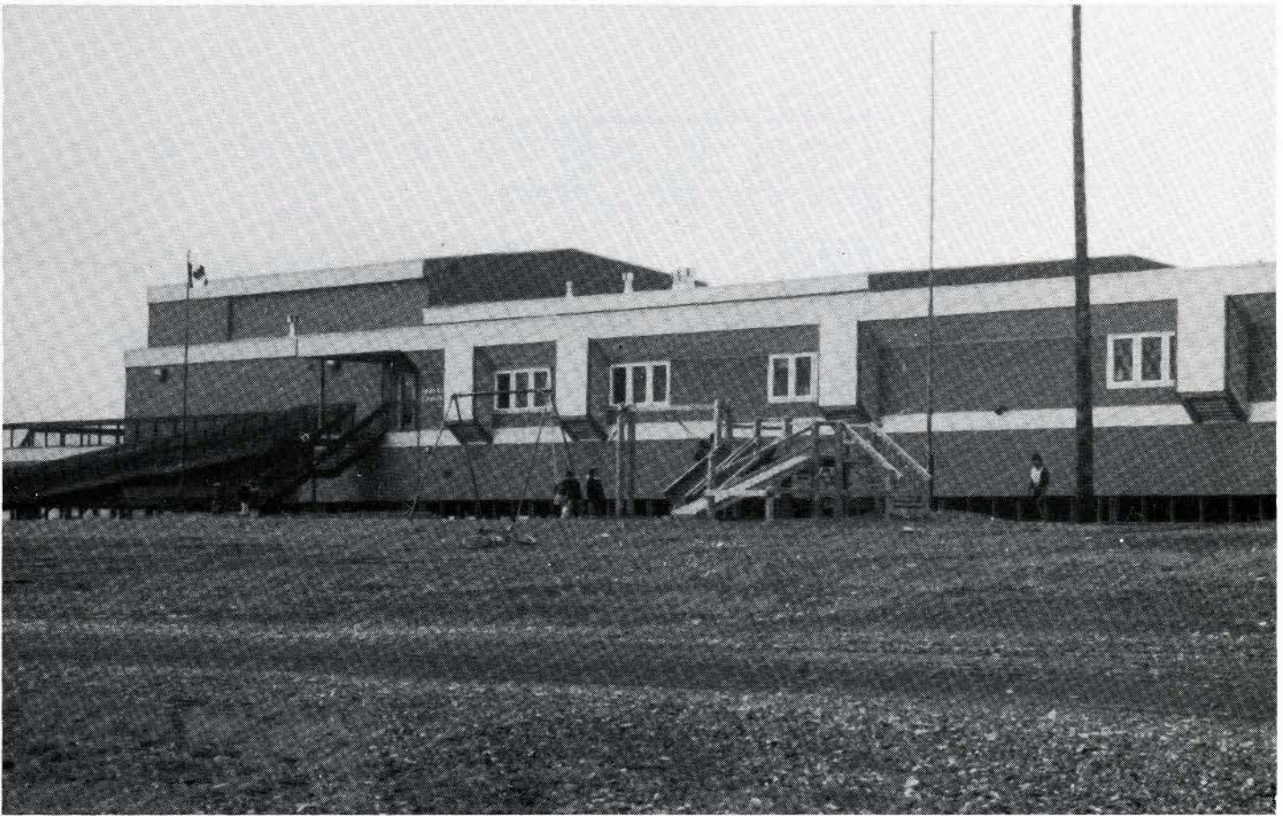
Figure 3. Homan School, Holman, NWT (1984). Exterior showing streamlined roof form and articulation of insulation of eave structure and snow control covers on ventilation panels.
