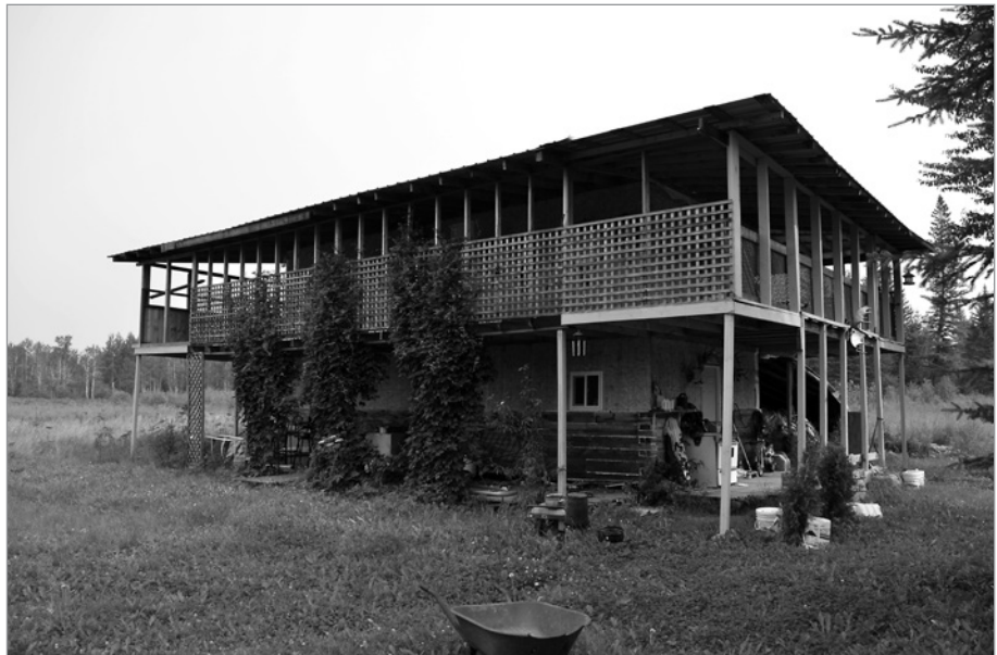
FIG. 4. EXTERIOR OF MUSKEG HOME, EAST PRAIRIE SETTLEMENT. | DAVID T. FORTIN.
