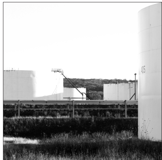
Refinery Tank Farm – 2015.
