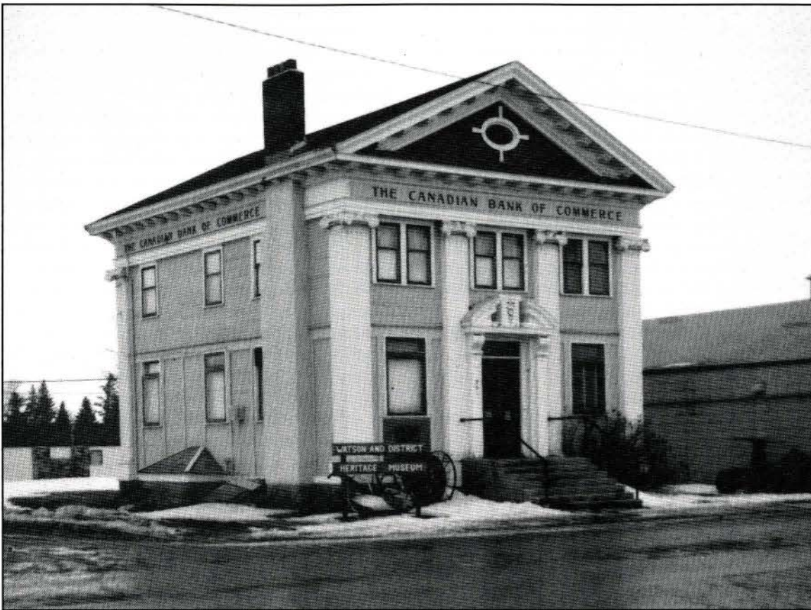
The pre-fabricated Beaux-Arts Canadian Bank of Commerce in Watson, Saskatchewan; Darling and Pearson, architects, 1906. (Environment Canada, Heritage Recording Services, 1990)
