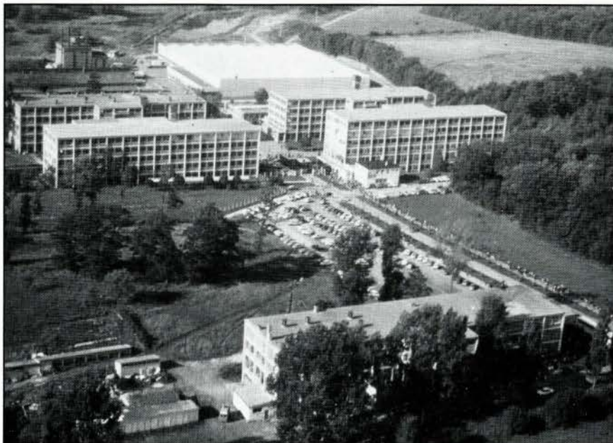
Figure 3. The Bata factories at Hellocourt, France, were built on the same modular plan as that at Batawa, Ontario, and other factories around the world. (Bata Canada, n.d.)
