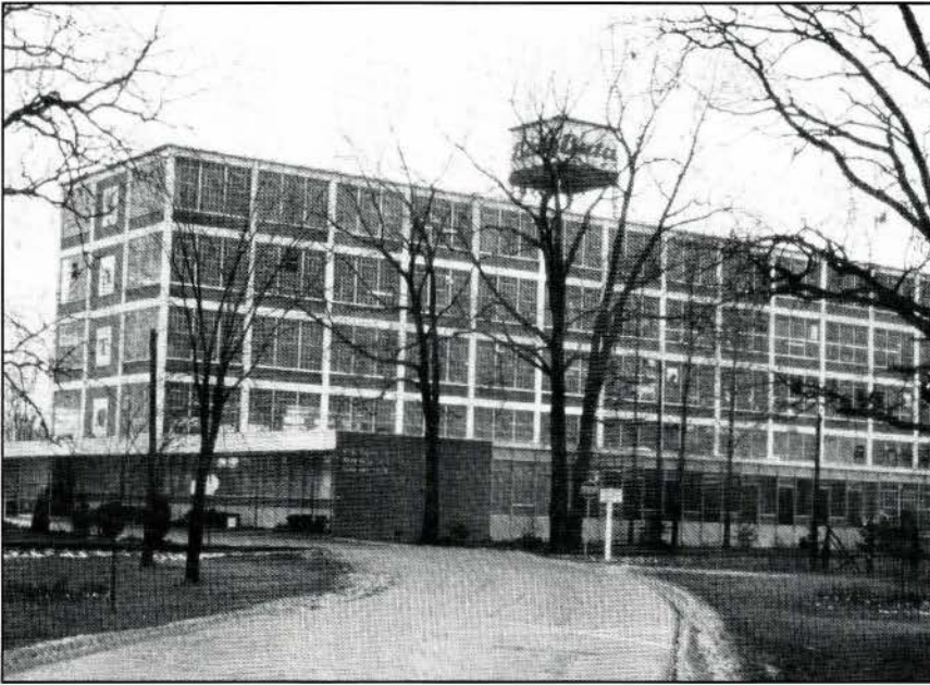
Figure 10 (left). The Bata factory at Batawa in the 1960s, before recladding. (Bata Canada)
