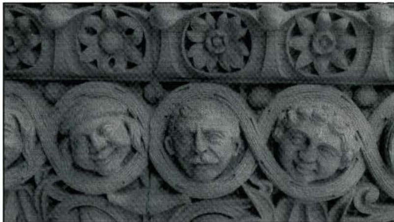
Column capital, Toronto City Hall.
