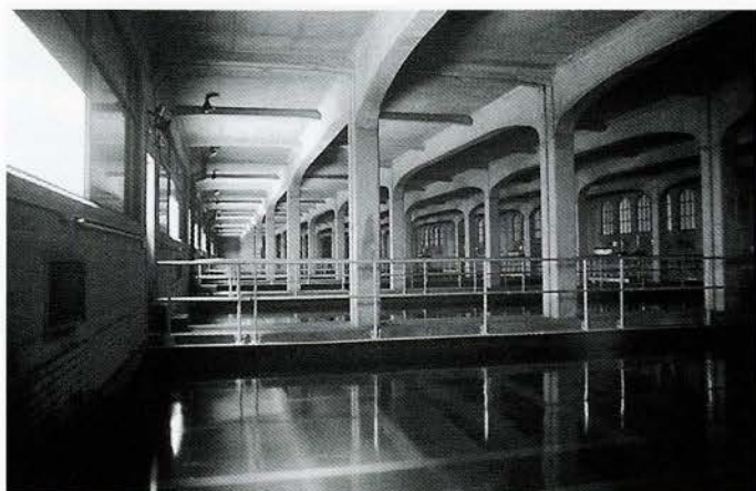
Fig. 9. View of filter bed, with glazed screen to filter gallery at right. (S. Mannell, 1998.)
