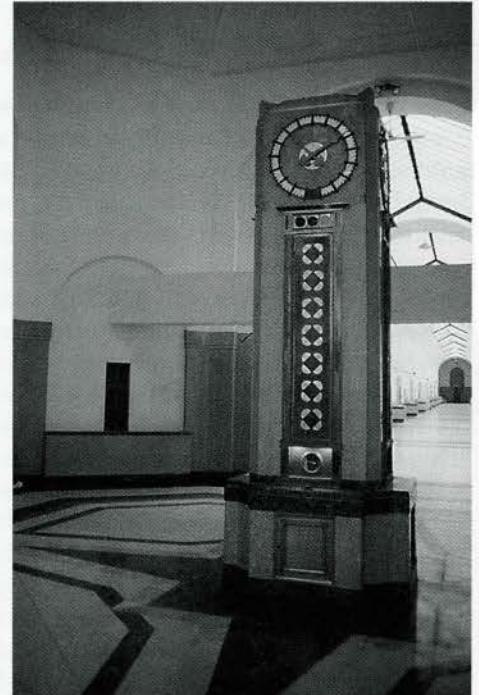
Fig. 7. Filter rotunda showing the signal pylon. (S. Mannell, 1997.)
