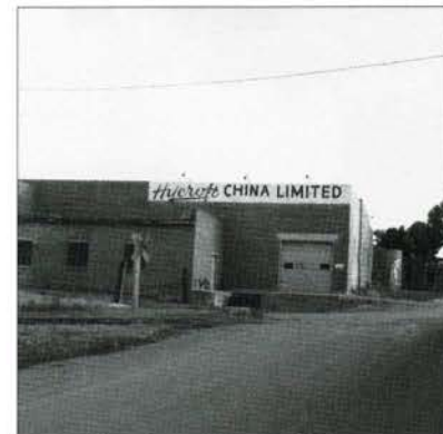
Fig. 13. View south to Hycroft complex from Wood Street entrance. (E. Mills, August 1999)
