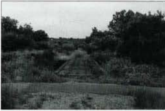
Fig. 27. View west along railway spur from trestle over Seven Persons Creek, midway between Medalta and the I-XL site. The track ends at this point. (E. Mills, August 1999)
