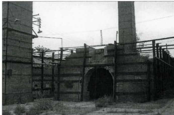
Fig. 33. Remnant of downdraft kiln associated with pre-1950 Medicine Hat Brick & Tile plant, I-XL complex. (Alberta Culture, Provincial Historic Resources Inventory , 1999)
