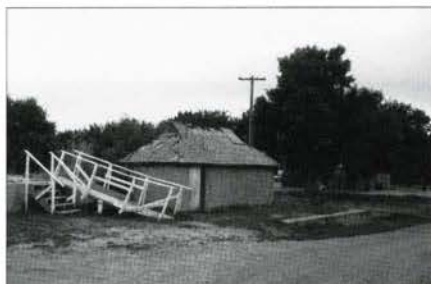
Fig. 11. Second gas regulator building at western perimeter of Hycroft Pottery site (brick regulator shed in background at right). (E. Mills, August 1999)
