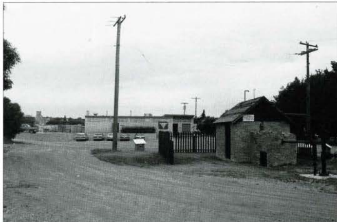
Fig. 10. View westward to Plainsman Clay Products factory entrance, with Alberta Clay Products gas regulator shed at right. (E. Mills, August 1999)
