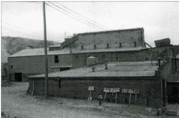
Fig. 32. Remnant of 1929 Medicine Hat Brick & Tile plant in I-XL complex. (Alberta Culture, Provincial Historic Resources Inventory , 1999)
