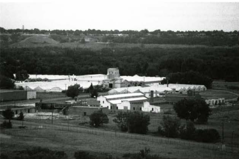
Fig. 3. Central section of proposed cultural landscape. National Porcelain site is in left foreground, Medalta Pottery in centre, commercial greenhouses in background. (E. Mills, August 1999)
