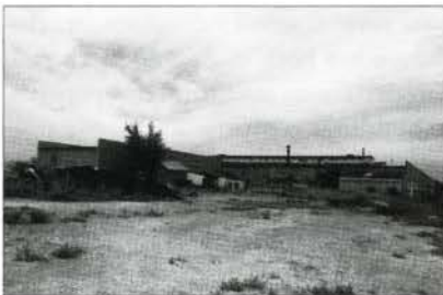
Fig. 16. Hycroft factory, eastern facade. (E. Mills, August 1999)
