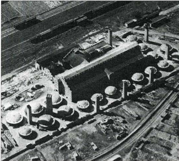
Fig. 6. Undated aerial view of Alberta Clay Products complex. CPR mainline is in background, spur line in lower foreground. The surviving beehive kiln appears at extreme left. (Marylu Antonelli and Jack Forbes, Pottery in Alberta. The Long Tradition , 34)
