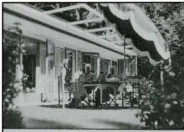
Fig. 18. Floor-to-ceiling glazed doors open onto the main terrace, extending the living-dining room into the garden. Comparison of the 1940s view (top) and the present-day view (bottom) reveals that very little has changed. (Photograph of c. 1948 slide belonging to Jessie Binning, documentation file, B.C. Binning Fonds, Collection Centre Canadien d'Architecture/Canadian Centre for Architecture, Montréal [top]; S.D. Bronson, September 1997 [bottom])
