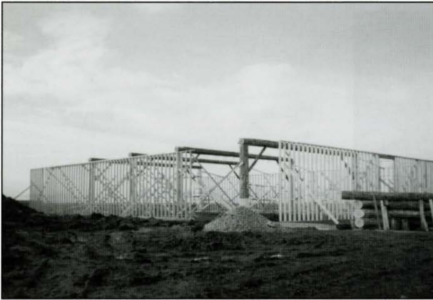
Fig. 2. Tsawwassen Longhouse under construction : a traditional post-and-beam structure. (Photo : Daniel Millette)
