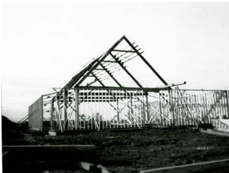
Fig. 1. Tsawwassen Longhouse under construction : the first frame pierces the second and reaches upwards to form a 12 metres high, pitched roof. (Photo : Daniel Millette)
