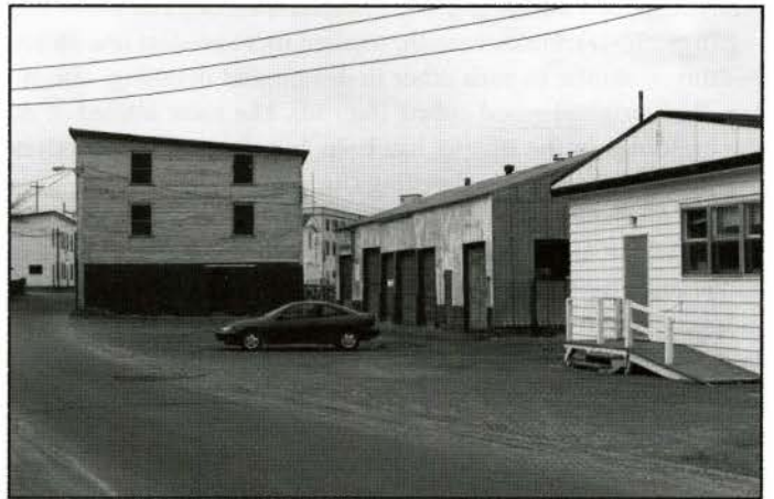
Fig. 42. View along main street, facing west, showing the side elevation of the factory, the 1930s garage and, on the far right, the former post office. (Photo: R. Goodspeed, HSB, 1998)
