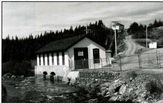
Fig. 7. Hydroelectric power station, with the Catalina River on the left and the flume on the right. The road to the immediate right of the flume, becoming a footpath further up, leads to the dams and reservoir higher up. (Photo: R. Goodspeed, HSB, 1998)
