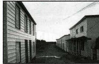
Fig. 16. View facing east along the upper road, showing the duplexes. The one on the right was built by a private individual. The intersection of that road with the one running southwest may be seen next to the first set of duplexes, 1997. (Ray Troke, Heritage Planner)
