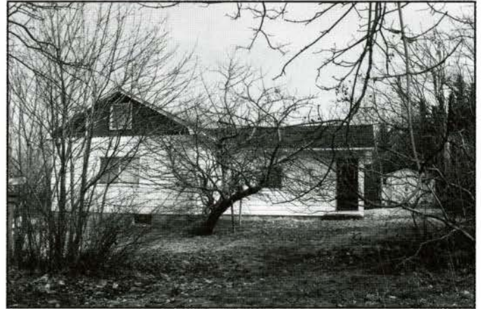
Fig. 40. Caretaker's house, beside the "Bungalow," ca. 1995-96. (Photo: R. Goodspeed, HSB, 1998)
