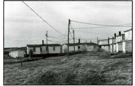
Fig. 47. Fields behind the houses above Bungalow Hill. The duplexes on the right are on the southwest side of the upper street.
