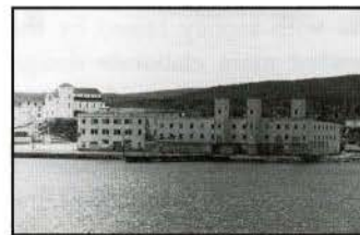
Fig. 25. Retail store on the left, fish plant on the right, and above Holy Martyrs Anglican Church, all built in 1946. (Photo: Ray Troke, Heritage Planner, ca. 1997)
