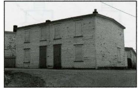
Fig. 50. A duplex from the upper street with no alterations. (Photo: R. Goodspeed, HSB, 1998)
