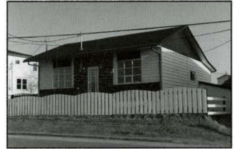
Fig. 51. The most altered of all the Coaker houses. (Photo: R. Goodspeed, HSB, 1998)
