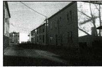
Fig. 15. View to the east of some of the houses along the lower, main street. The two in the distance originally had bay windows, while the vacant lot between two houses was previously the site of a duplex. On the right is the very edge of the front of the Coaker property. (Photo: R. Goodspeed, HSB, 1998)
