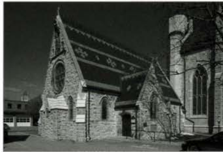
FIG. 3. KINGSTON, ST. JAMES BOANARGES CHAPEL. EXTERIOR. | MALCOLM THURLBY
