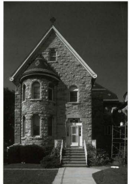
FIG. 44. GANANOQUE, ST JOHN THE EVANGELIST, RECTORY, EXTERIOR FROM E. | MALCOLM THURLBY
