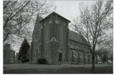
FIG. 14. PRESCOTT, ST. MARK. EXTERIOR FROM SW (SE). | MALCOLM THURLBY
