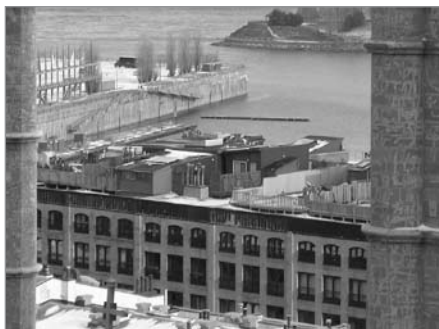
FIG. 16. MONTREAL'S HABITABLE ROOF AT COURS LE ROYER, 1981, DESNOYERS MERCURE GAGNON AND SHEPPARD ARCHITECTS. | ALENA PROCHAZKA.
