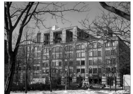
FIG. 20. CLOS SAINT-BERNARD RENOVATION BY DAN S. HANGANU, 1986. | PIERRE BOYER-MERCIER.
