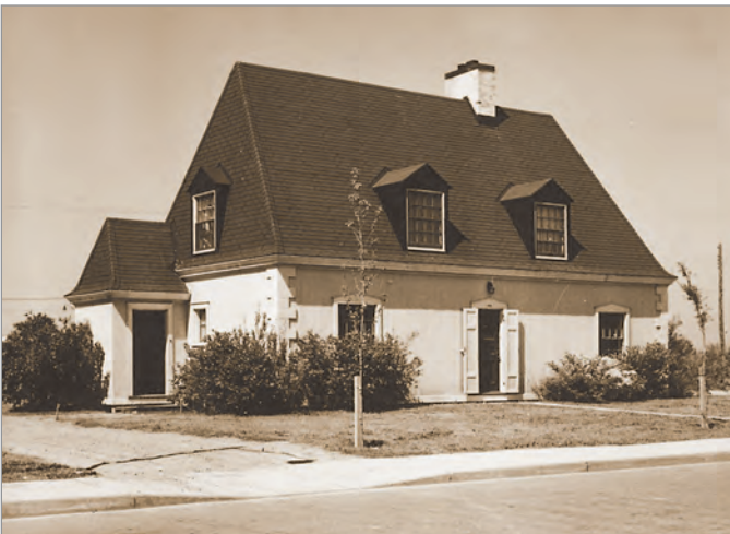
FIG. 56. THE REGIONALIST FIGURATION OF THIS HOUSE, BUILT IN ARVIDA IN 1942, EARNED IT AND MANY OF ITS ARVIDA SIBLINGS A PLACE IN INVENTAIRE DES ŒUVRES D'ART DU QUÉBEC , UNDER THE HEADING "MODERN RESIDENCE IN THE FRENCH CANADIAN STYLE." | SYLVIO BRASSARD, INVENTAIRE DES ŒUVRES D'ART DU QUÉBEC , 1944, BIBLIOTHÈQUE ET ARCHIVES NATIONALES DU QUÉBEC.
