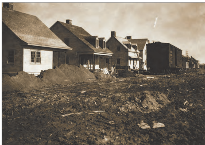
FIG. 63. CONSTRUCTION SITE OF THE "CITY BUILT IN 135 DAYS." A RAILCAR DISTRIBUTES PRECUT ARCHITECTURAL COMPONENTS FROM LOT TO LOT. | SOCIÉTÉ HISTORIQUE DU SAGUENAY.
