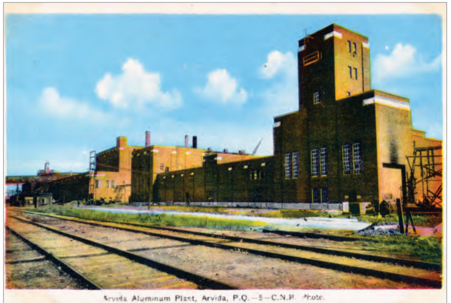
FIG. 35. THE ARVIDA BAUXITE REFINERY, OR SLAG ORE PLANT, WAS PROMOTED ON POSTCARDS FROM ITS INAUGURATION IN 1927. IN LIGHT OF UNSATISFACTORY RESULTS FROM THE INITIAL DRY PROCESS, A BAYER PROCESS REFINERY WAS BROUGHT ON LINE TO REPLACE IT IN 1935, WITH PLANS BY ARCHITECT J.C. MEADOWCROFT. | BIBLIOTHÈQUE ET ARCHIVES NATIONALES DU QUÉBEC.
