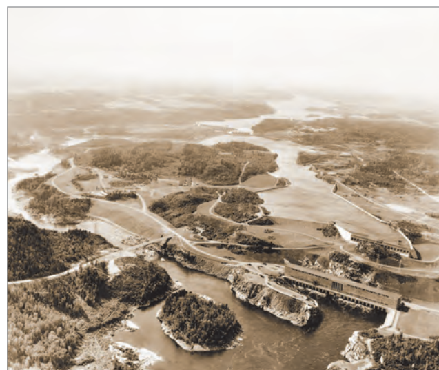
FIG. 33. THE SAGUENAY RIVER HYDROELECTRIC FACILITIES AROUND 1952. PLANS DATE BACK TO 1925 FROM THE ALUMINUM COMPANY OF AMERICA AND WERE COMPLETED BY THE ALUMINUM COMPANY OF CANADA WITH THE INAUGURATION OF THE SHIPSHAW II POWER PLANT AND DAM (FOREGROUND) IN 1942. THE FIRST OF THE TWO PLANTS, CHUTE-À-CARON, WITH ITS GRAVITY DAM, PUT INTO OPERATION IN 1931, IS SEEN IN THE BACKGROUND UPSTREAM. THE TWO SPECTACULAR PROJECTS SUCCESSIVELY CREATED THE MOST POWERFUL GENERATING STATION IN THEIR RESPECTIVE DAYS. | LIBRARY AND ARCHIVES CANADA.
