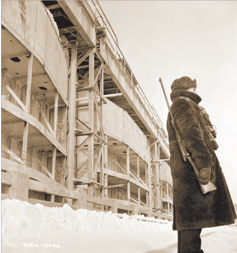
FIG. 70. ARMED GUARD BY THE SHIPSHAW DAM. THE POWER STATION WAS BUILT IN BARELY 18 MONTHS IN 1942, STILL ACCORDING TO THE 1925 HYDROELECTRIC DEVELOPMENT PLANS. THE DAM, SMELTER, REFINERIES, AND CITY OF ARVIDA TOOK ON STRATEGIC IMPORTANCE TO THE COMMONWEALTH DURING THE SECOND WORLD WAR, AND EXCEPTIONAL MEASURES WERE TAKEN TO PROTECT THEM, INCLUDING CONSTRUCTION OF ANTI-AIRCRAFT BATTERIES AND THE ESTABLISHMENT OF THE BAGOTVILLE MILITARY BASE. | LIBRARY AND ARCHIVES CANADA.
