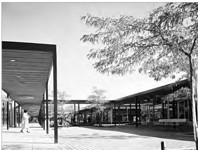
FIG. 4. JOHN B. PARKIN ASSOCIATES, DON MILL SHOPPING CENTRE 1953-1955, VIEW OF THE MAIN MALL. | CANADIAN ARCHITECTURAL ARCHIVES LIBRARY AND CULTURAL RESOURCES, PANDA COLLECTION: PAN 59963-48.
