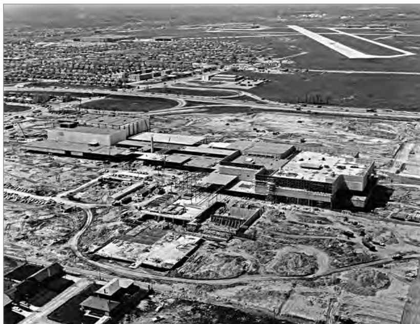
FIG. 9. JOHN B. PARKIN ASSOCIATES, JOHN GRAHAM CONSULTANTS LTD., VICTOR GRUEN ASSOCIATES, YORKDALE SHOPPING CENTRE, 1962-1964, CONSTRUCTION SITE, CA. 1962, WITH HIGHWAY 401 AND DOWNSVIEW AIRPORT IN THE BACKGROUND. | CANADIAN ARCHITECTURAL ARCHIVES AND CULTURAL RESOURCES, PANDA COLLECTION: PAN 63379-1.
