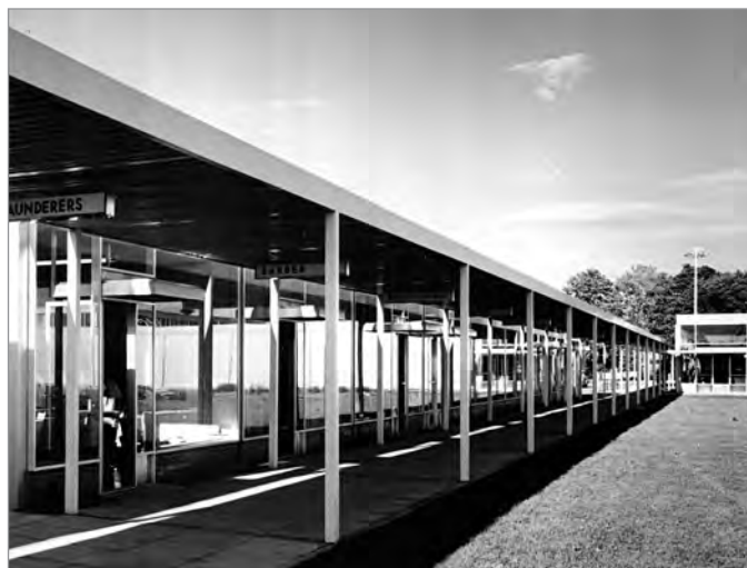
FIG. 5. DON MILL SHOPPING CENTRE, 1953-1955, VIEW OF THE ROW OF SHOPS. | CANADIAN ARCHITECTURAL ARCHIVES AND CULTURAL RESOURCES, PANDA COLLECTION: PAN 55943-19.
