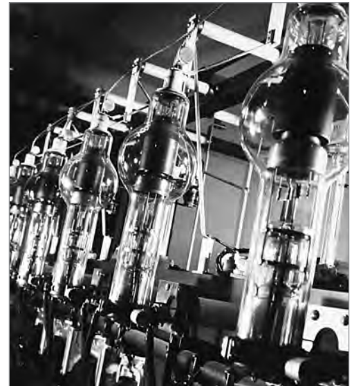
FIG. 11. PART OF THE BANK OF HIGH VOLTAGE RECTIFIER TUBES WHICH CHARGE THE ALTERNATING CURRENT SUPPLIED BY HYDRO INTO A DIRECT CURRENT SUPPLY REQUIRED FOR THE OPERATION OF THE VACUUM TUBES IN THE 50,000-WATT TRANSMITTER. | CANADIAN BROADCASTING CORPORATION FONDS, LIBRARY AND ARCHIVES CANADA, RG 41, VOL. 542 FILE PART 1, E010934711.
