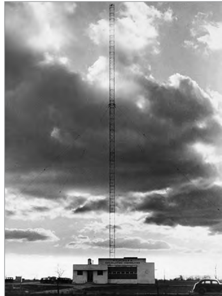
FIG. 6. CBL BUILDING AND TOWER DURING CONSTRUCTION, 1937. | CANADIAN BROADCASTING CORPORATION FONDS, LIBRARY AND ARCHIVES CANADA, RG 41, VOL. 542 FILE PART 1, E010934714.
