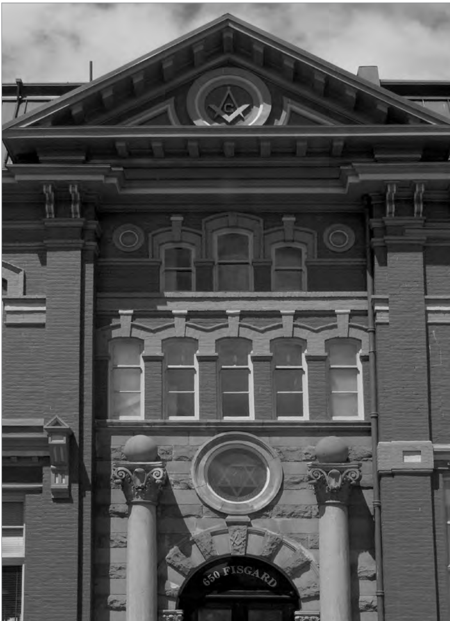
FIG. 1. MASONIC LODGE, 650 FISGARD STREET, VICTORIA, BRITISH COLUMBIA, 1878-1908. | PIERRE DU PREY, 2012.
