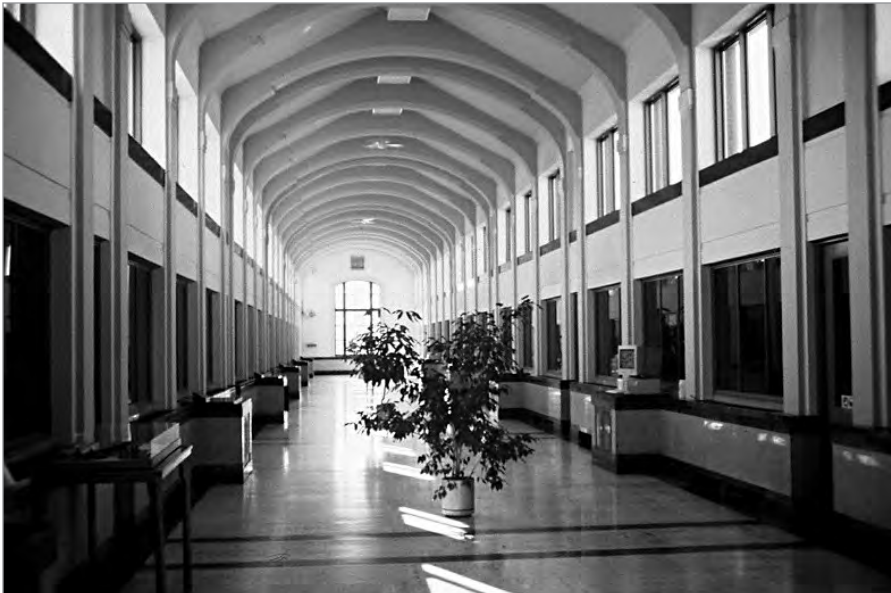
FIG. 17. LEMIEUX ISLAND WATER WORKS, OTTAWA, 1932. VIEW OF THE FILTER GALLERY SHOWING GLAZED SCREENS ENCLOSED THE FILTER BEDS. THE PILASTERS EXTEND THROUGH THE ROUND ARCHES AT THE PORTAL FRAMES TO CREATE AN INTEGRATED RHYTHM. FLOORS AND WAINSCOT ARE MARBLE AND TRAVERTINE. | STEVEN MANNELL, 2001.
