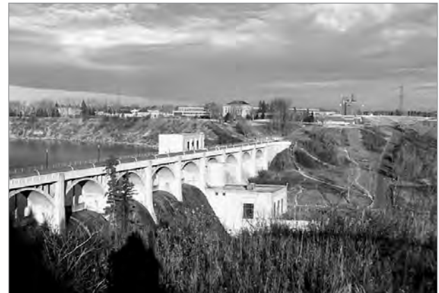
FIG. 12. GLENMORE WATER WORKS, CALGARY, 1934. VIEW OF THE DAM AND BRIDGE, WITH THE WATERWORKS BUILDINGS BEYOND. | STEVEN MANNELL, 2001.
