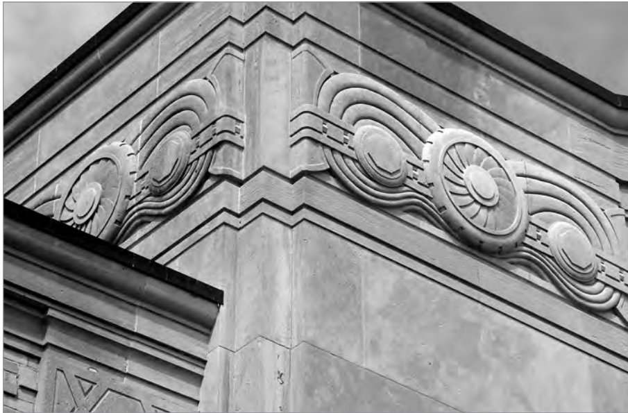
FIG. 31. VICTORIA PARK WATER WORKS. VIEW OF CORNER PILASTER AT THE PUMPING STATION SHOWING THE TURBINE CAPITAL. | LAUREEN VAN LIEROP, 2010.
