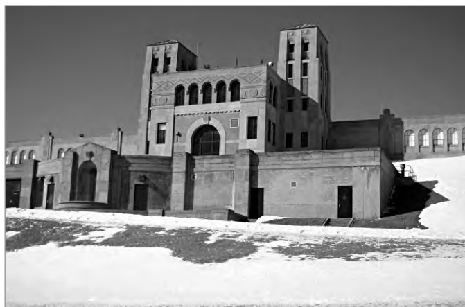
FIG. 30. VICTORIA PARK WATER WORKS. VIEW FROM THE SOUTH OF THE TERRACE SHOWING THE GROTTA AND FOUNTAIN AS BUILT; BEYOND IS THE TRIUMPHAL ARCH FORM OF THE ADMINISTRATION AND FILTER BUILDING ENTRANCE, FLANKED BY PAIRED TOWERS. THE ROUND ARCHES OF THE GROTTA AND THE ENTRY SHARE A CONSOLE KEYSTONE PROFILE. | STEVEN MANNELL, 2008.
