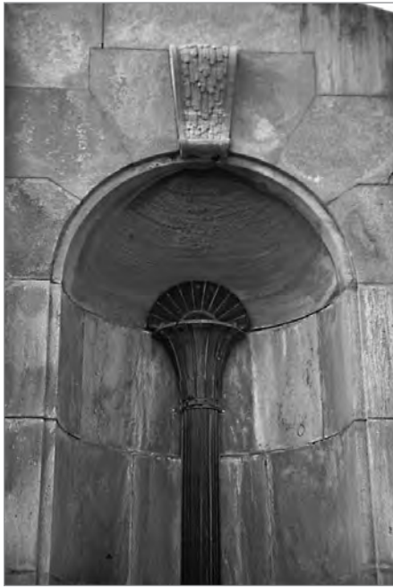
FIG. 36. VICTORIA PARK WATER WORKS. DETAIL OF ARCH, KEYSTONE, AND BRONZE FOUNTAIN AT THE SOUTH FAÇADE OF THE TERRACE. | STEVEN MANNELL, 1998.
