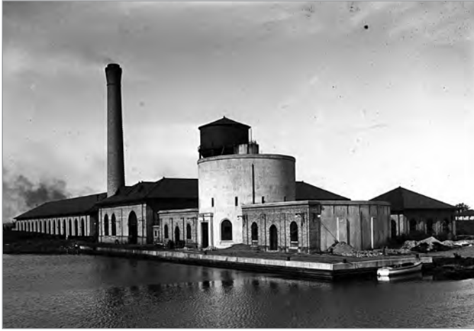
FIG. 7. OVERALL VIEW OF THE DRIFTING-SAND FILTRATION PLANT AT CENTRE ISLAND, AUGUST 27, 1918. THE STUCCO CYLINDER HOUSES CHEMICAL STORAGE, WITH A FAN OF CHEMICAL FEED BASINS IN THE LOW ROUND BUILDING AT ITS BASE. BEYOND ARE THE PUMPING STATION, THEN THE SMOKESTACK FOR ITS COAL-FIRED POWER GENERATORS FOR THE PUMPS, AND FINALLY THE LONG FILTER BUILDING. | ARTHUR GOSS. CTA, SERIES 372, SUBSERIES 72, ITEM 897.
