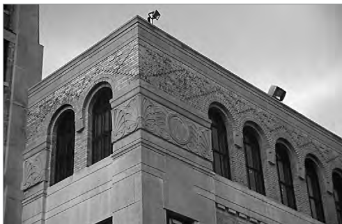
FIG. 29. VICTORIA PARK WATER WORKS. DETAIL OF CORNER PILASTER AT THE ADMINISTRATION WING SHOWING THE FOLDED SCALLOP SHELL CAPITALS CROWNING THE STONE PILASTERS. | STEVEN MANNELL, 1998.
