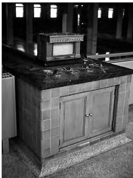
FIG. 15. GLENMORE WATER WORKS. VIEW OF THE FILTER GALLERY SHOWING THE ABSENCE OF GLAZED SCREENS TO THE FILTER BEDS, AND THE TERRAZZO, TILE AND PLASTER FINISH PALETTE. THE DECORATION OF THE CEILING IS ONLY LOOSELY RELATED TO THE ORDER OF THE WALL SURFACES. | STEVEN MANNELL, 2001.
