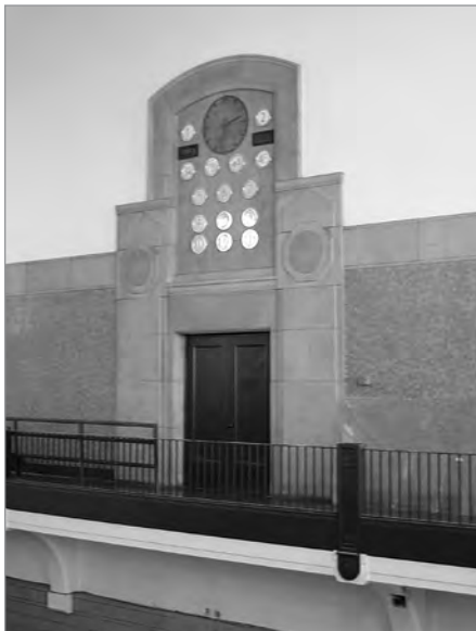
FIG. 33. VICTORIA PARK WATER WORKS. VIEW OF THE SIGNAL PANEL IN THE PUMPING STATION. THE LIGHTS INDICATE WHICH FILTERS ARE IN OPERATION, WHILE THE DIAL INDICATES WATER FLOW. | STEVEN MANNELL, 2010.
