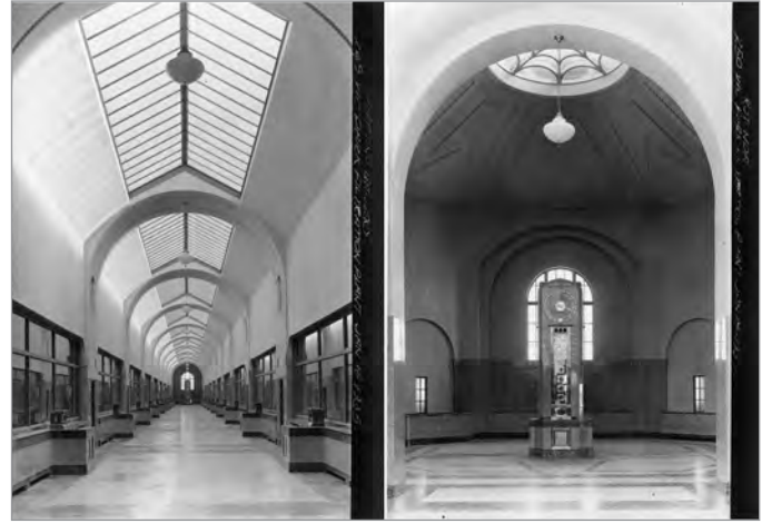
FIG. 3. INTERIOR VIEWS OF THE COMPLETED ADMINISTRATION AND FILTER BUILDING AT VICTORIA PARK, JANUARY 18, 1935, SHOWING THE WEST FILTER GALLERY LOOKING TOWARD THE FILTER ROTUNDA (LEFT), AND THE FILTER ROTUNDA (RIGHT) SHOWING THE MARBLE SIGNAL PYLON THAT BROADCASTS INFORMATION ABOUT THE PURIFICATION PROCESS. | ARTHUR GOSS, TORONTO WATER.
