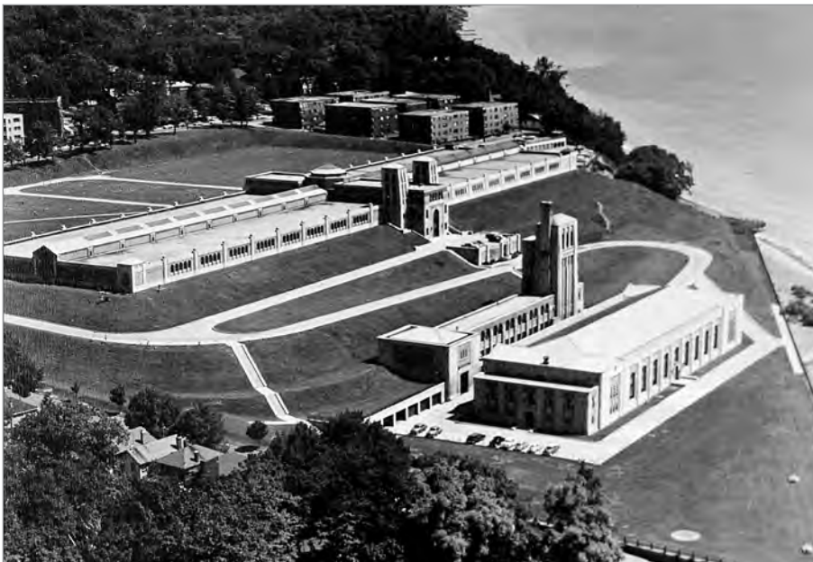
FIG. 1. TORONTO WATER WORKS EXTENSION - VICTORIA PARK WATER WORKS (NOW THE R.C. HARRIS WATER TREATMENT PLANT), AERIAL VIEW FROM THE SOUTHWEST. THE ADMINISTRATION AND FILTER BUILDING IS AT THE TOP OF THE SLOPE, WITH THE ADMINISTRATION WING IN THE CENTRE BETWEEN THE PAIRED TOWERS, AND THE TERRACE AND FOUNTAIN IN FRONT. THE SERVICE BUILDING IS EMBEDDED IN THE SLOPE, WITH THE ALUM TOWER EMERGING AT THE EAST END, PROVIDING A BACKDROP TO THE FREESTANDING TEMPLE VOLUME OF THE PUMPING STATION. | CITY OF TORONTO ARCHIVES (CTA), PUBLIC WORKS COLLECTION, SERIES 160.
