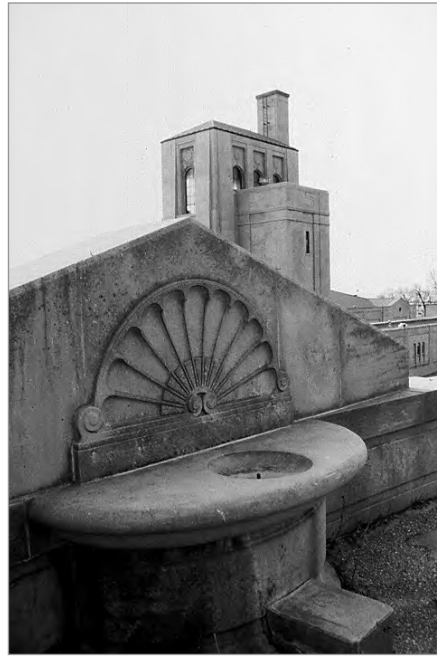
FIG. 37. VICTORIA PARK WATER WORKS. DRINKING FOUNTAIN ON THE TOP OF THE TERRACE LOOKING TOWARD THE ALUM TOWER AND THE LAKE. | STEVEN MANNELL, 1998.
