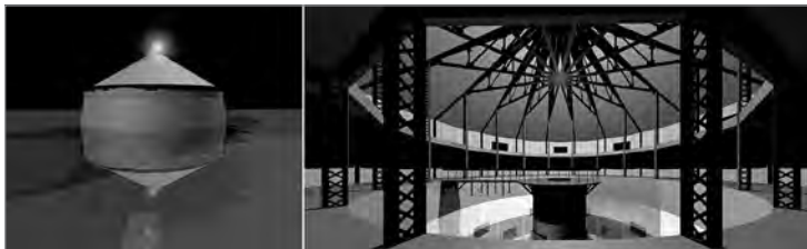
FIG. 10. RECONSTRUCTION OF THE OFFSHORE INTAKE CRIB OF THE 1913 DESIGN FOR THE VICTORIA PARKS WATER WORKS SHOWING THE EXTERIOR AT NIGHT (LEFT), AND THE INTERIOR WITH THE UPPER LEVEL ACCESS GALLERY TO CREW'S QUARTERS (RIGHT). | DIGITAL MODELS AND RENDERINGS BY STEVEN MANNELL AND CHAD JAMIESON, 2003.
