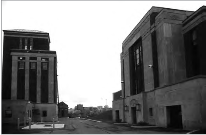
FIG. 19. LEMIEUX ISLAND WATER WORKS. VIEW OF THE MAIN DRIVEWAY, FRAMED BY THE ADMINISTRATION AND FILTER BUILDING TO THE RIGHT, AND THE ALUM TOWER TO THE LEFT. | STEVEN MANNELL, 2001.
