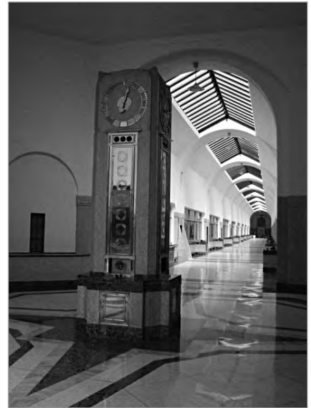
FIG. 32. VICTORIA PARK WATER WORKS. VIEW OF THE SIGNAL PYLON, WITH MARBLE OPERATING TABLES AND GLAZED SCREENS TO THE FILTER BEDS. | STEVEN MANNELL, 2010.
