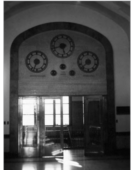
FIG. 18. LEMIEUX ISLAND WATER WORKS. VIEW OF THE FILTER GALLERY SIGNAL PANEL, ABOVE THE DOORS TO THE ADMINISTRATION WING. | STEVEN MANNELL, 2001.
