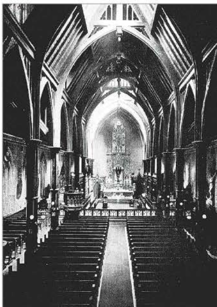
FIG. 16. ST. BASIL'S CATHOLIC CHURCH, TORONTO, ARCHIVAL PHOTOGRAPH – INTERIOR LOOKING EAST. | COURTESY OF THE UNIVERSITY OF ST. MICHAEL'S COLLEGE ARCHIVES.
