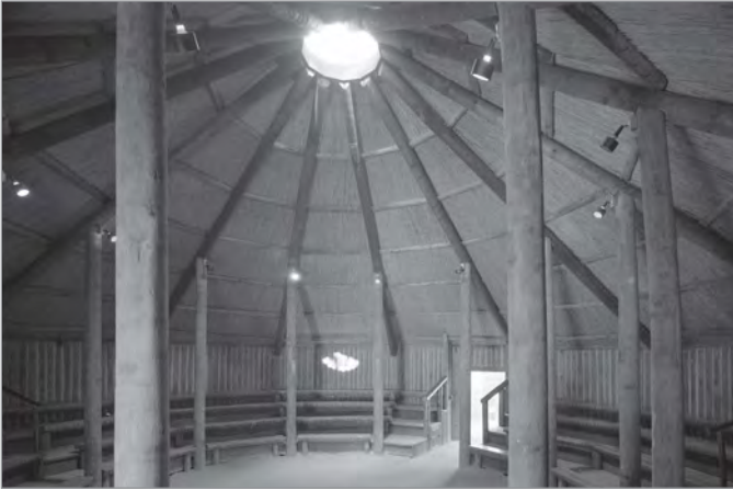
FIG. 12. BARRY MORE. ALABAMA COUSHATTA MUSEUM AND VILLAGE. CEREMONIAL BUILDING. 1972. PHOTO: RICK GARDNER. COURTESY HOUSTON PUBLIC LIBRARY, HMRC, MSS 0078-3615. | HOUSTON PUBLIC LIBRARY, HMRC, MSS 0078-3615.
