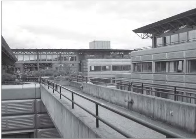
FIG. 4. FROM HIS INTERNATIONAL SURVEY, BANHAM OMITTED THE ÉCOLE POLYTECHNIQUE FÉDÉRALE DE LAUSANNE (EPFL) (ZWEIFEL AND STRICKLER, 1970-1982), ALONG WITH OTHER SIGNIFICANT CONTRIBUTIONS TO THE LEGACY OF THE MEGASTRUCTURE MOVEMENT SUCH AS LETHBRIDGE UNIVERSITY (ERICKSON MASSEY, 1969-1971) AND ONTARIO PLACE (CRAIG ZEIDLER AND STRONG, 1968-1971), PERHAPS BECAUSE HE HAD STARTED LOSING INTEREST BY 1973, OR EVEN EARLIER. | JAMES ASHBY.
