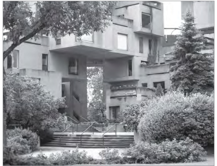
FIG. 7. HABITAT '67 (MOSHE SAFDIE WITH DAVID, BARROTT, BOULVA, 1962-1967) IS EXCEPTIONAL AMONG CANADIAN MEGASTRUCTURES IN ITS DESIGNATION AS MONUMENT HISTORIQUE CLASSÉ (2009). | JAMES ASHBY.
