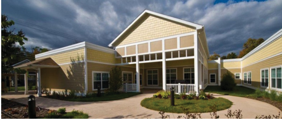
Figure 49: The addition of the RK MacDonald Nursing Home in Antigonish Nova Scotia, an Eden Alternative Home. (RK MacDonald Nursing Home 2007)
