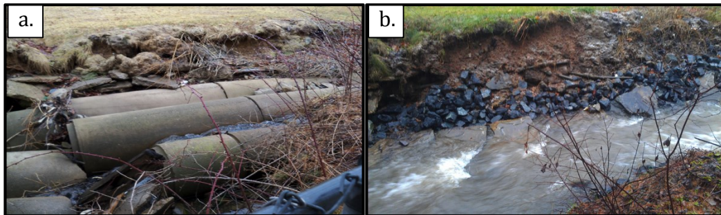
Figure 4.2: Culverts in a feeder brook a) pre-removal, and b) post-removal.
