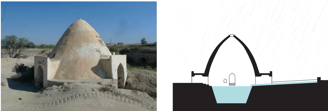
Figure 56: Rainwater Collection Cistern
