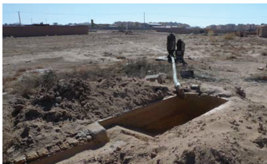
Figure 87: Small agricultural pump Agricultural pumps usually feature a pool in which the water is poured and the sediments allowed to settle before the water reaches its destination.
