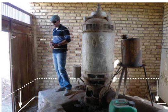
Figure 88: Large agricultural pump A significant amount of land subsidence is visible in the image above. Due to the continuous extraction of water, the pumphouse building has dropped nearly 100cm below its original foundation over the course of several years.
