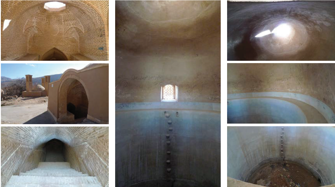
Figure 27: Interior and exterior of Ab Anbars, made with bricks. The interior of reservoir is lined with sarooj , a specially formulated water resistant plaster. The exterior brick is sometimes left exposed and sometimes covered with a clay and straw compound called kah-ghel . (photos from 2014)
