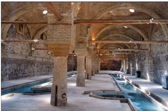
Figure 63: Rakhtshooy Khaneh (Laundry Washing House)
