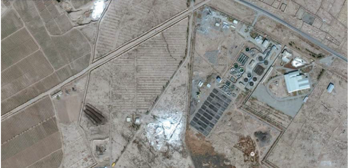
Figure 94: Sewage Treatment Plant
