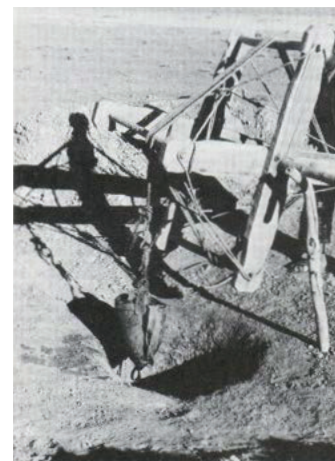
Figure 154: A winch bringing the spoil to the surface. (Wulff 1966)
