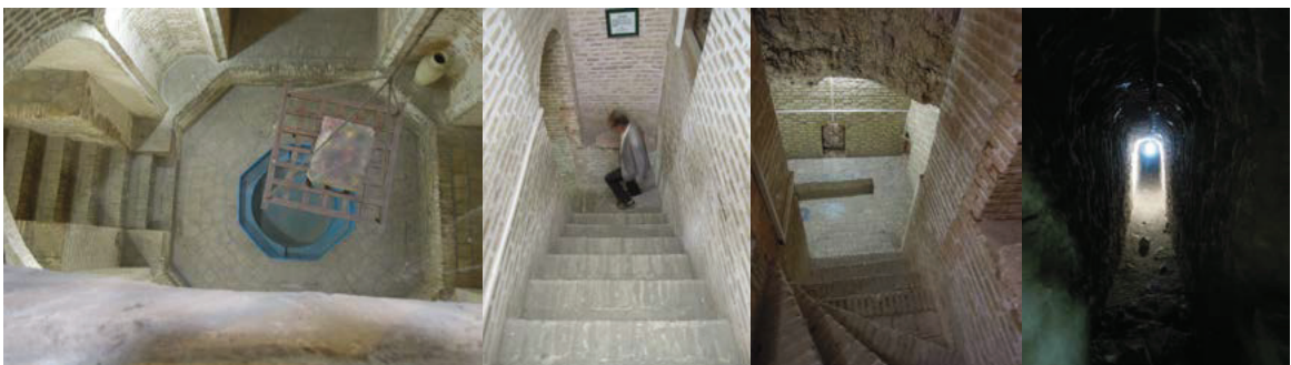
Figure 54: Private residential payab accessed below grade due to cool temperatures in the summer.
