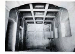
Fig. 14: The windtower room of the Gazorgh house. Note the twelve openings from the windtower.
