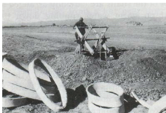
Figure 156: Qanat-lining hoops. (Wulff 1966)
