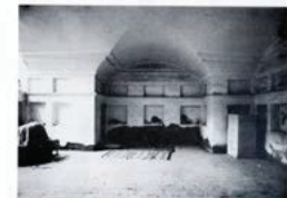
Fig. 15: The main underground room beneath the iwan of the Gazorgh house. Light is coming from the elevation on the upper left.
