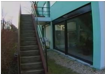
Quartier Modern Fuges restored to original condition (Brand 1994)
