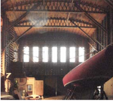
Belfast trusses in Snyder's Shipyard
