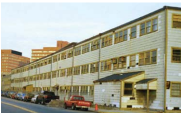
Building 20 shortly before demolition. (Molloy 2013)
