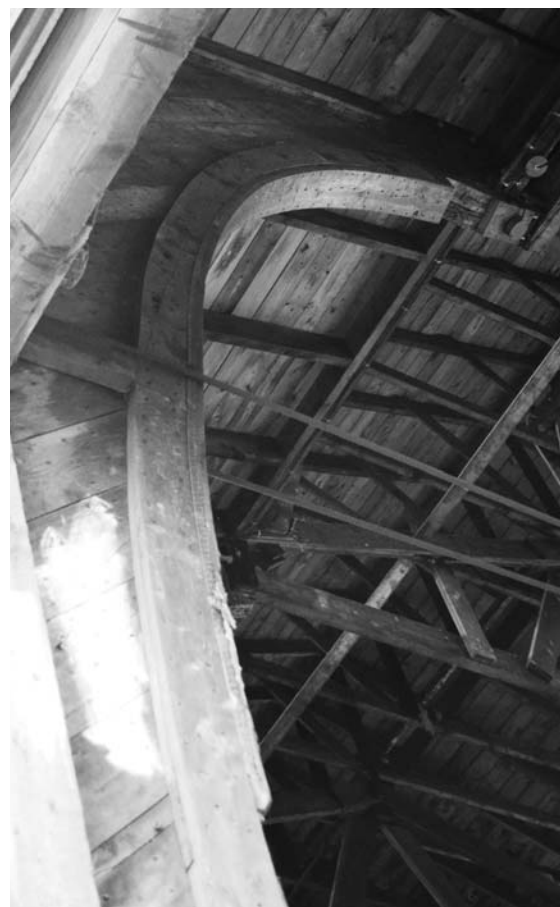
Arched bracing Bluenose shed
