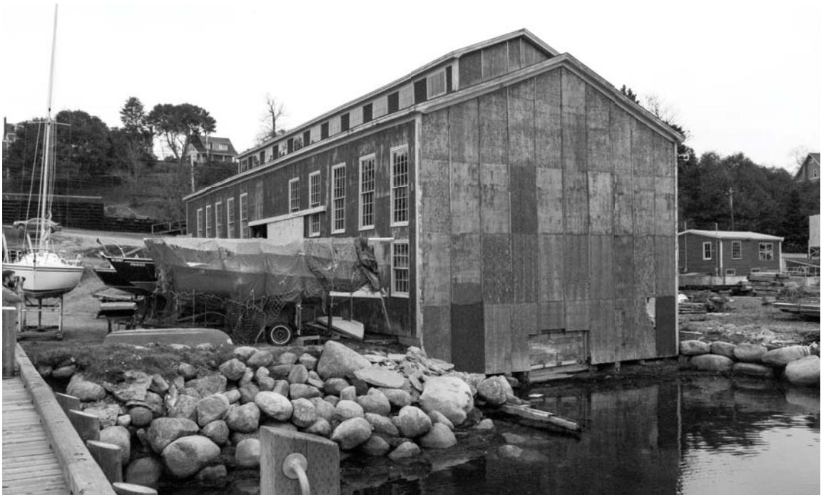
Bluenose shed - note exterior wall clad with plywood
