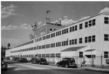
Building 20 shortly after construction. (Magical Incubator, MIT Video 1998)
