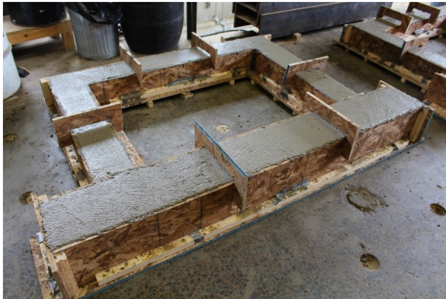
Figure 3.8 Completion of concrete casting
