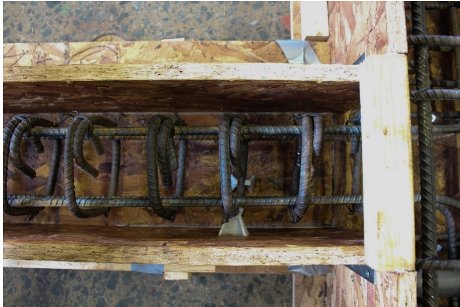
Figure 3.6 Details of formwork with reinforcement
