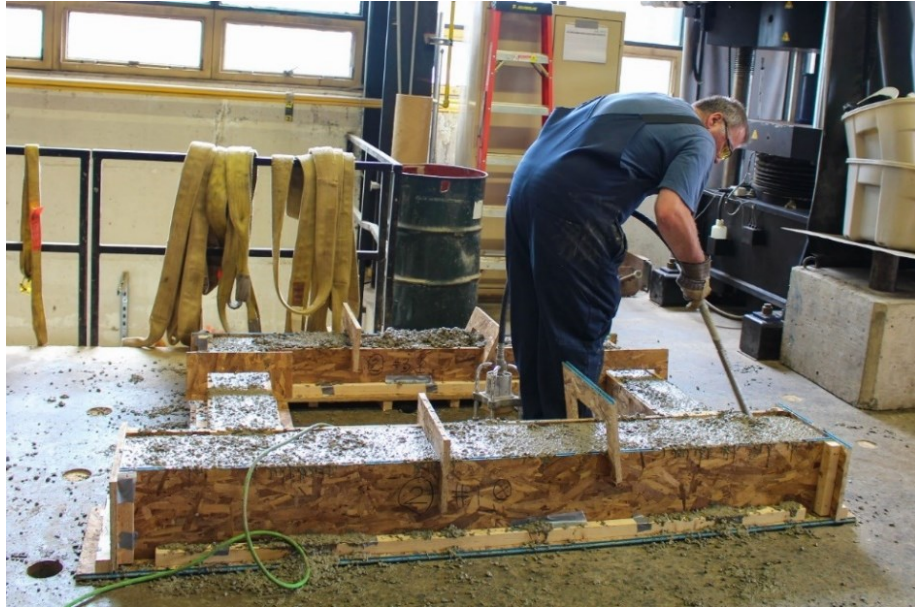
Figure 3.7 Concrete casting and vibrating
