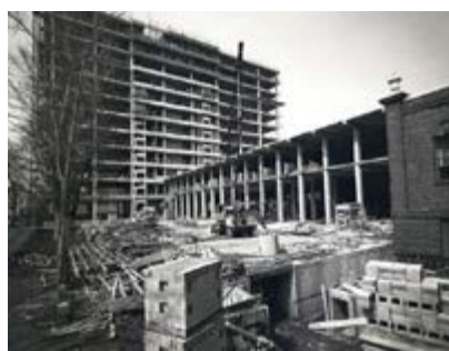
Tupper Building construction, n.d.
