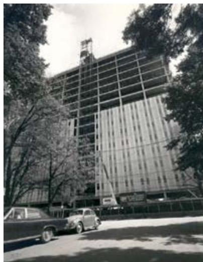
Tupper Building construction, n.d.
