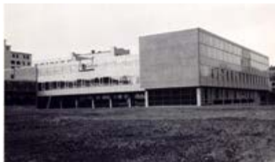
Administration and CAD/CAM Centre - Exterior, n.d.
