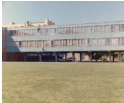
Administration and CAD/CAM Centre - Exterior - Side View, n.d.
