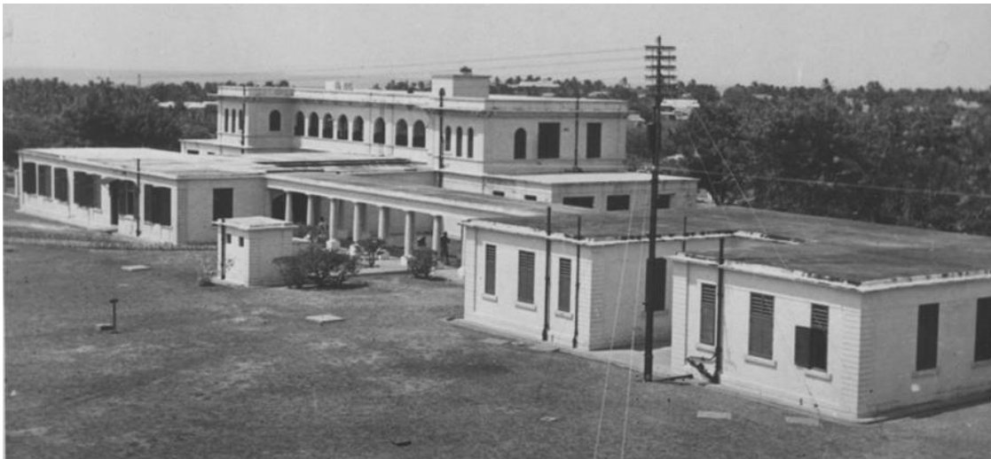
Figure 5.3. Rear view of the out-patients department, which included the X-ray, eye and dental sections, of the Gold Coast Hospital, circa 1940. Evident here are the power lines, which brought electricity from a generator on the campus to provide power for the machinery and lights in the hospital. Source: Basel Mission Archive Photo, ref #: QD-30.102.0001.
