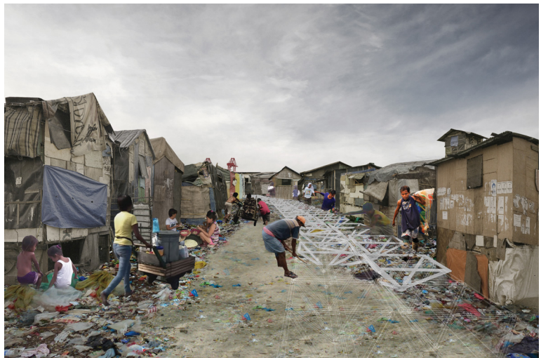
Figure 107: Space frame utilidor being constructed by the residents
