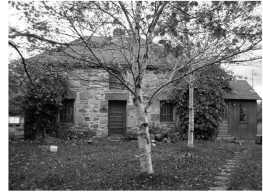
Front elevation, MacRae-Bitterman House, Middle River, Cape Breton, NS, 2004, photographer unknown (Nova Scotia Dept. of Tourism, Culture and Heritage 2004)
