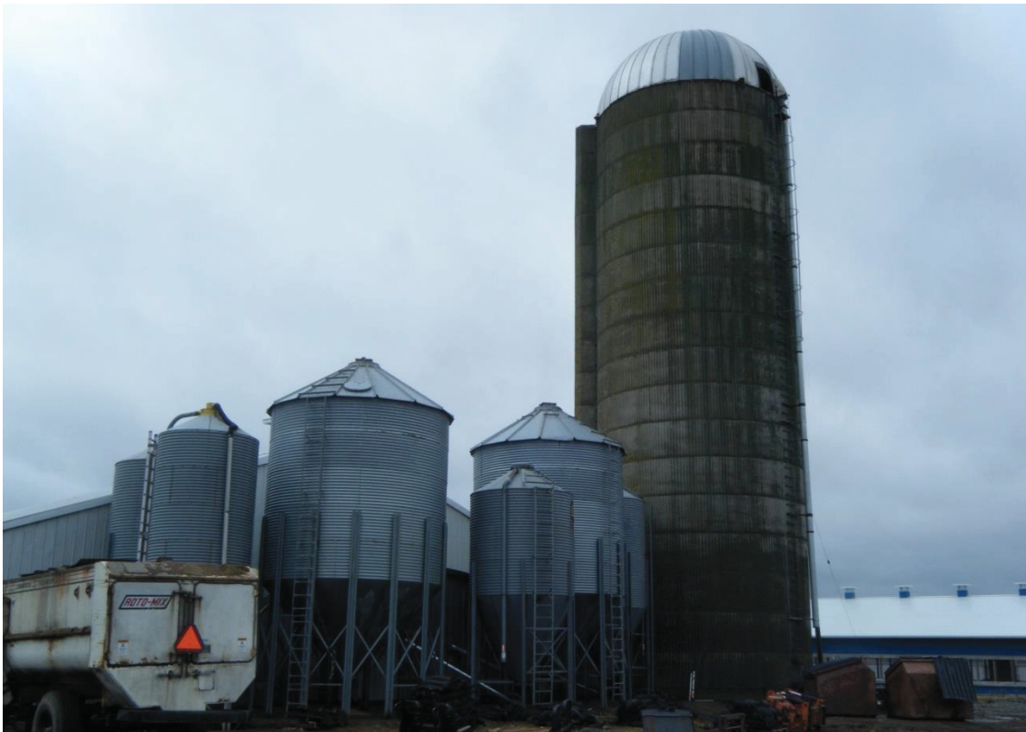
Figure 12: Tower silo and Bins
