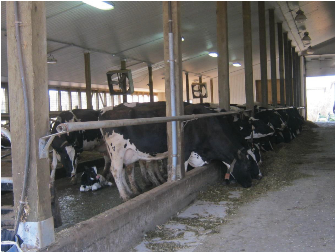
Figure 11: Natural ventilation with cooling fans in one of the audited dairy farm
