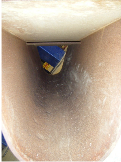
Figure D.37: Specimen C2 inside of stiffening rib.
