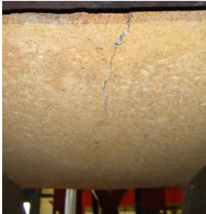
Figure 7.15: Specimen A3 failure due to pitting corrosion of deck plate.
