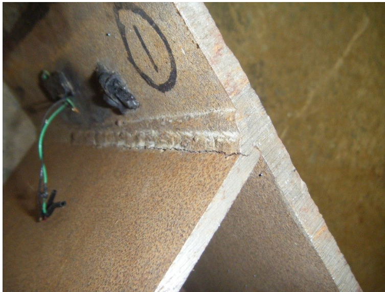
Figure 7.11: Root-weld cracking on Specimen A21.
