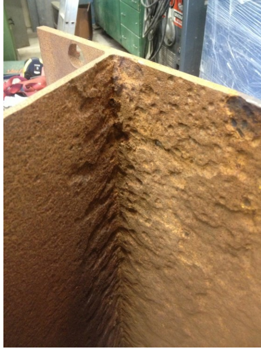
Figure D.35: Specimen C5 deck to stiffening rib connection.
