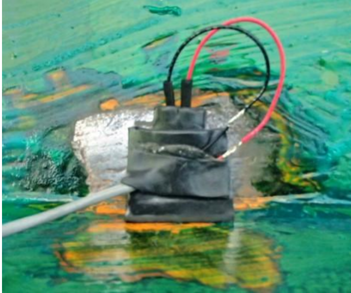
Figure A.5: Type A gauge before application of waterproofing membrane (courtesy of KTM).
