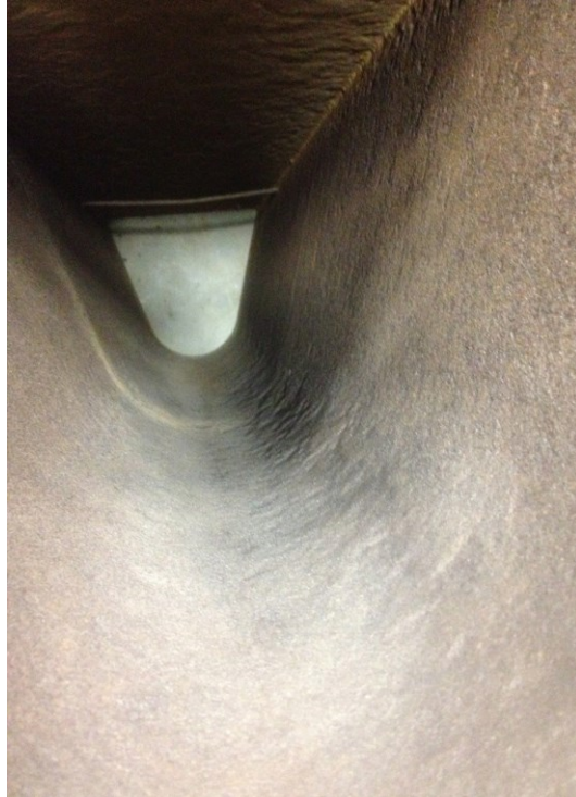
Figure D.33: Specimen C4 bottom of stiffening rib.
