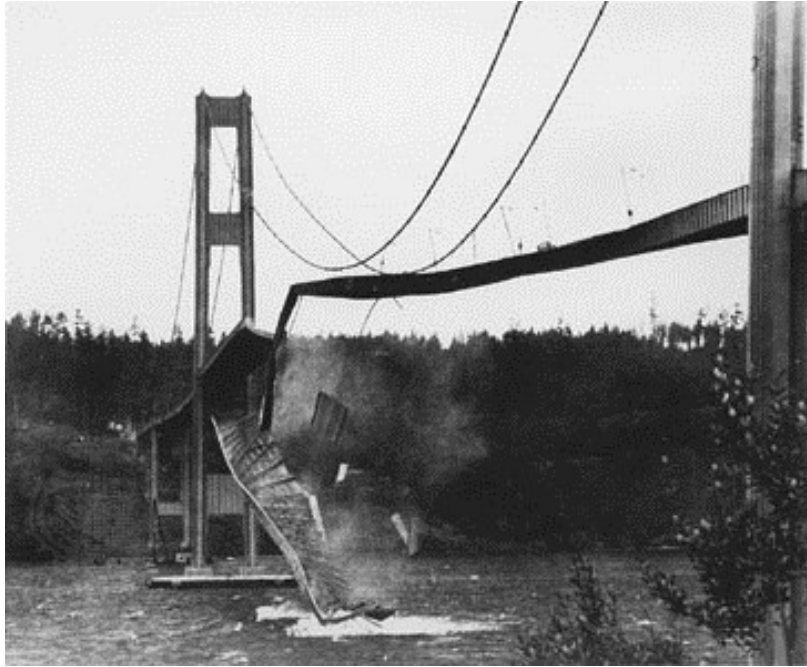
Figure 2.3: Tacoma Narrows during collapse, 1940 (Blockley 2010)
