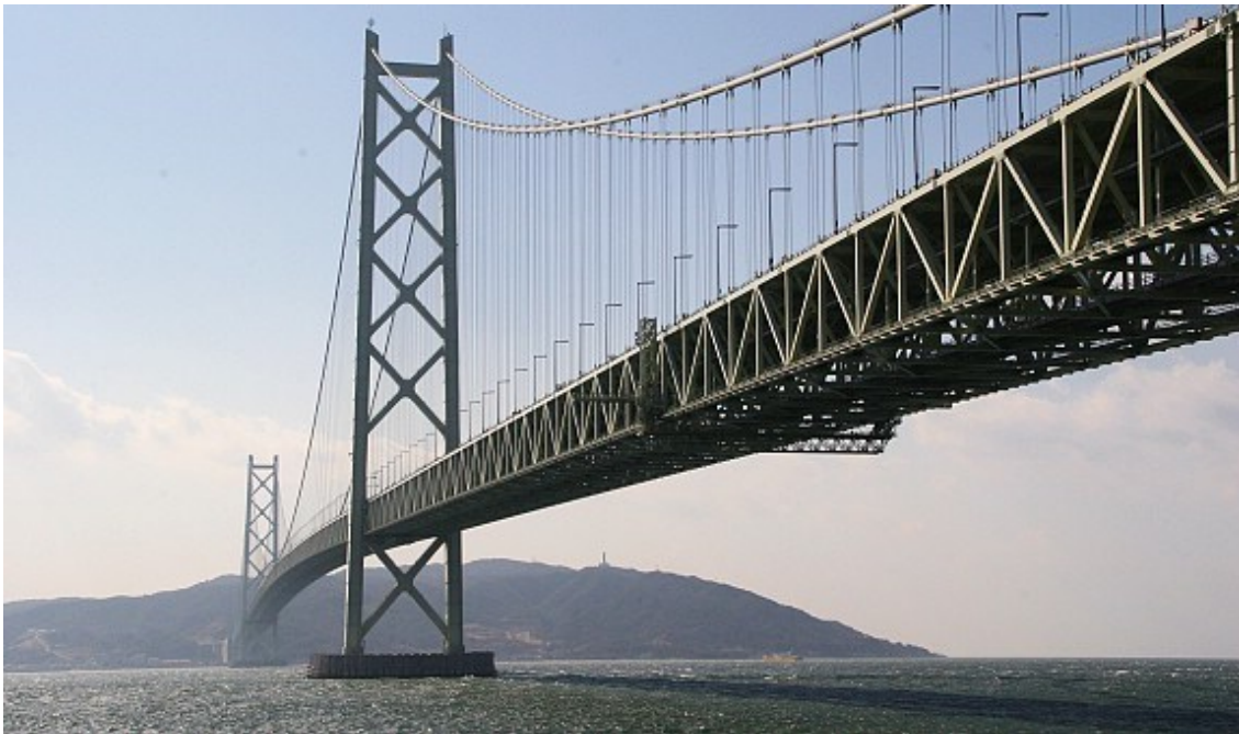
Figure 2.4: The Akashi Kaikyō Bridge, Japan (Kawada 2010)
