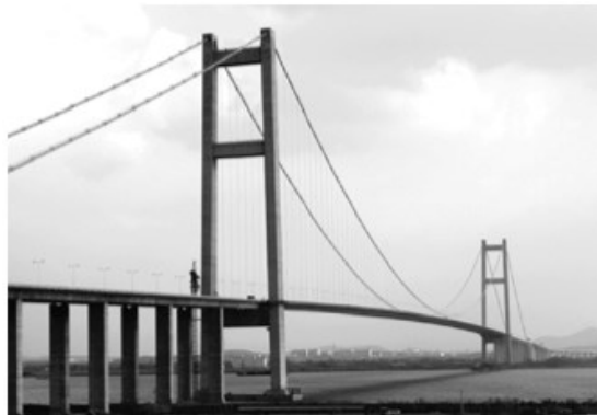
Figure 2.9: Runyang Suspension Bridge (Miao et al. 2013)
