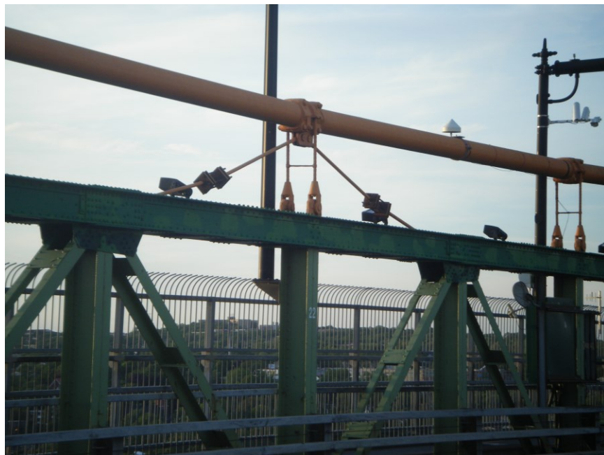
Figure 3.9: Traction rods for Main Span
