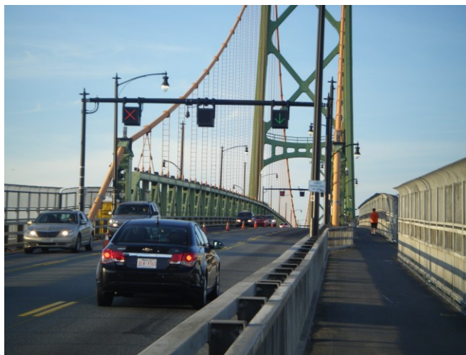
Figure 3.1: Alternating center lane, Halifax approach span looking towards Dartmouth
