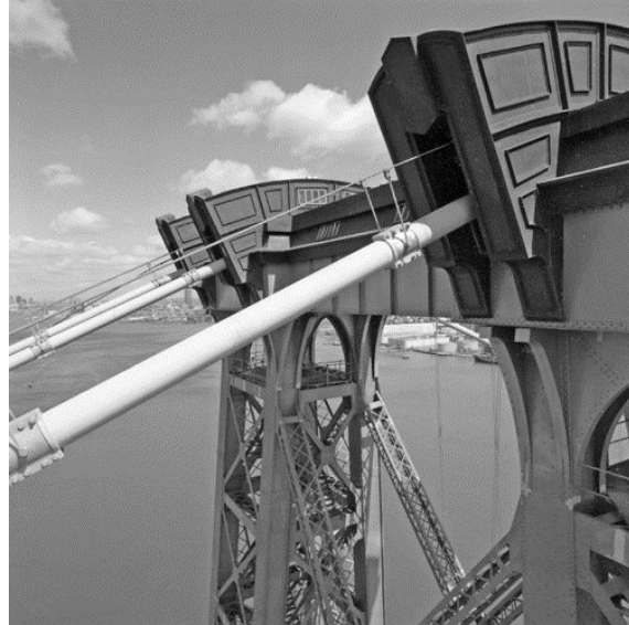
Figure 2.6: Cable saddles atop main towers, Williamsburg Bridge (ICE 2008)
