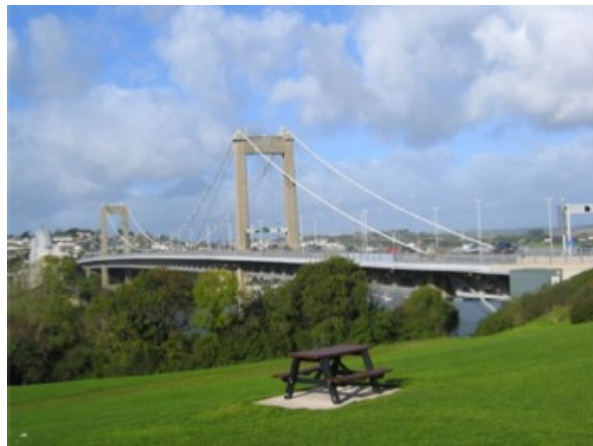
Figure 2.11: Tamar Suspension Bridge (Battista et al. 2011)
