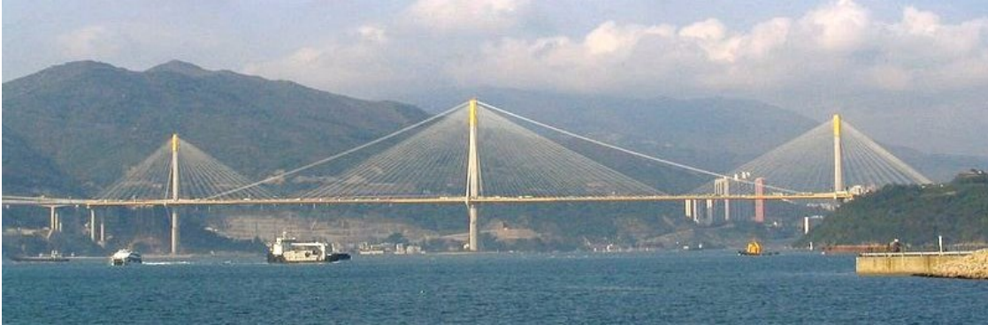
Figure 2.10: Ting Kau Bridge
