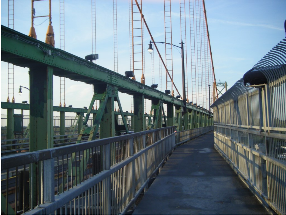
Figure 3.7: Stiffening truss, looking towards Dartmouth from walkway
