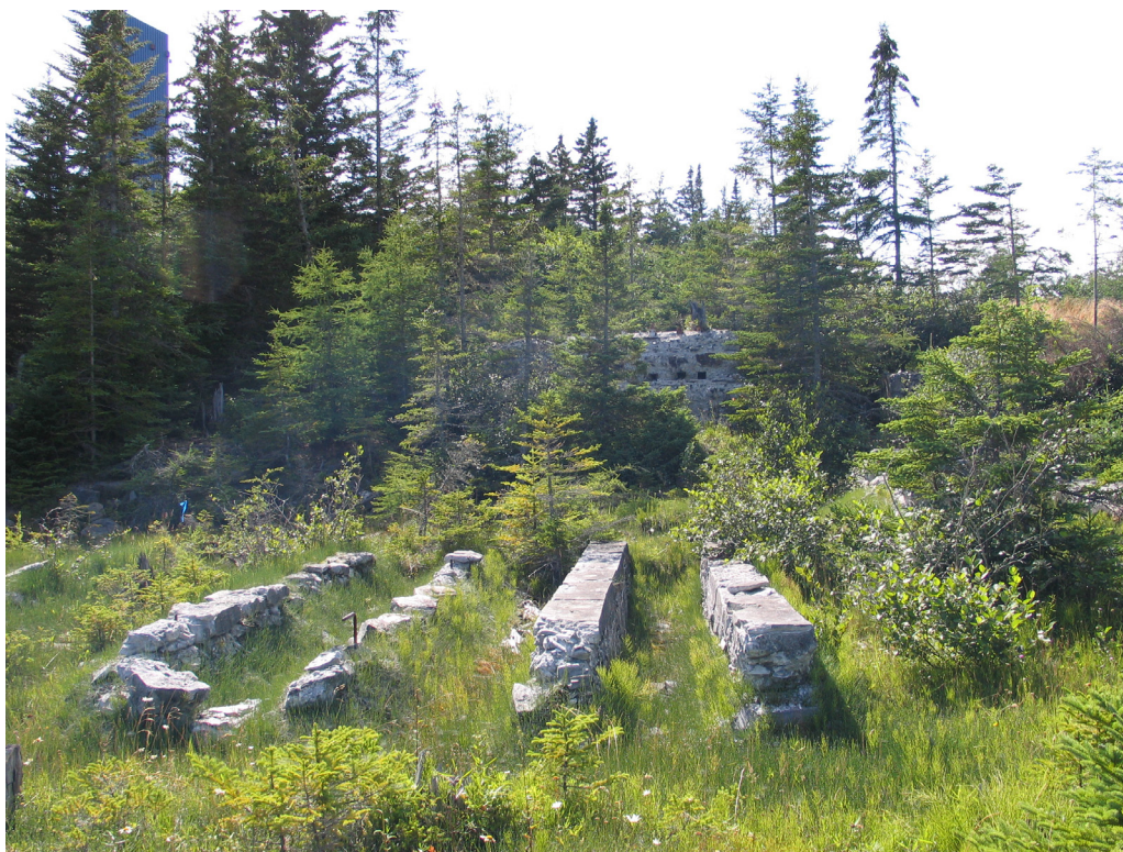
Figure 39 Deteriorating cement foundations and rotted timbers are all that remain of the massive Richardson Mill building complex located on the southwestern shore of Gold Brook Lake. The Boston Richardson head frame (rebuilt in the 1980s) can be seen in the upper left.
