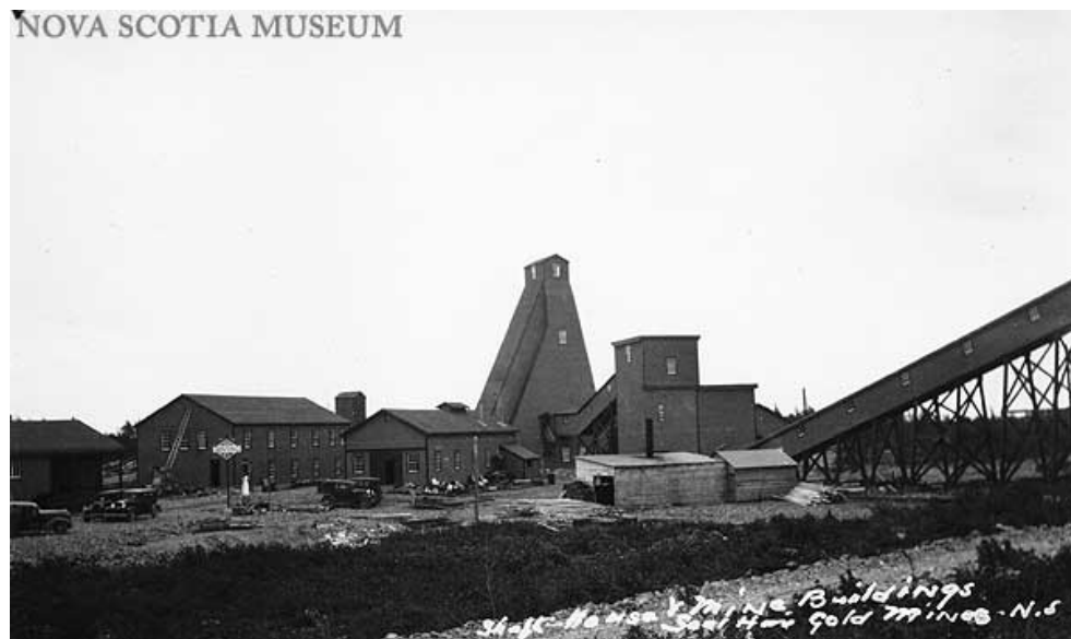
Figure 41. (a) View of stamps at the Dolliver Mountain Mine, ca. 1902. These were transported to the Lower Seal Harbour district in 1905. Photo taken by E.R. Faribault, Geological Survey of Canada. Reproduced with permission from the Earth Sciences Sector Photo Library Collection, Natural Resources Canada, Ottawa; (b) Shaft house, mine buildings, crusher, and ore conveyer leading to the cyanide plant at the Lower Seal Harbour Mine, ca. 1937 (Nova Scotia Museum of Cultural History Photo P270.286).
