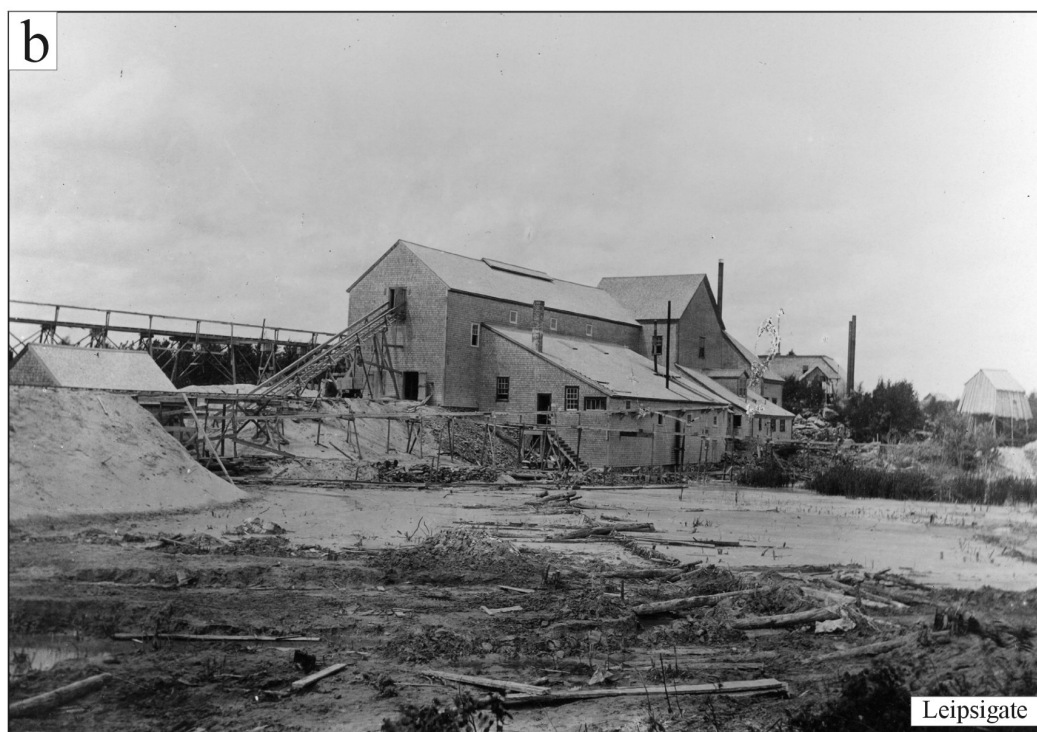
Figure 3. Unconfined tailings disposal from stamp mills at the (a) Mooseland, and (b) Leipsigate gold mining districts in 1897 and 1904, respectively. Photos taken by E.R. Faribault, Geological Survey of Canada. Reproduced with permission from the Earth Sciences Sector Photo Library Collection, Natural Resources Canada, Ottawa.
