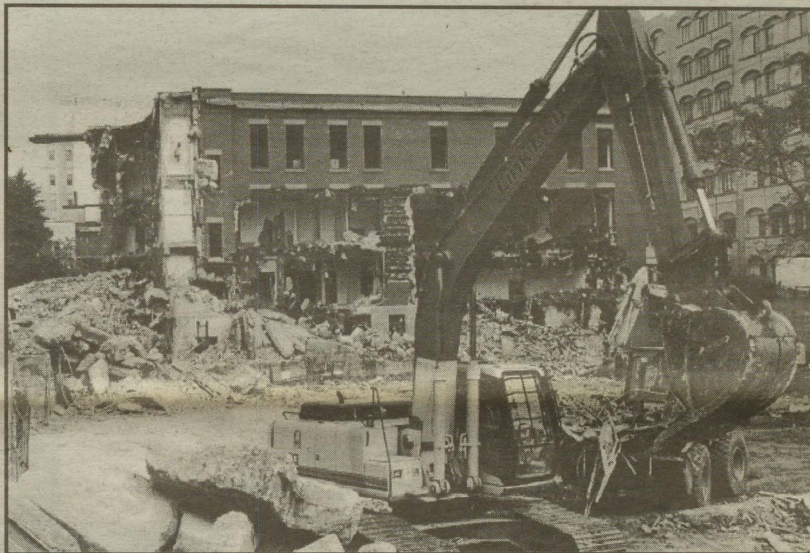
A backhoe picks up wreckage from the old Halifax Civic Building adjacent to the IWK Hospital. Crews have been tearing down the building for the past few weeks. Photo by Luke Dobek.
